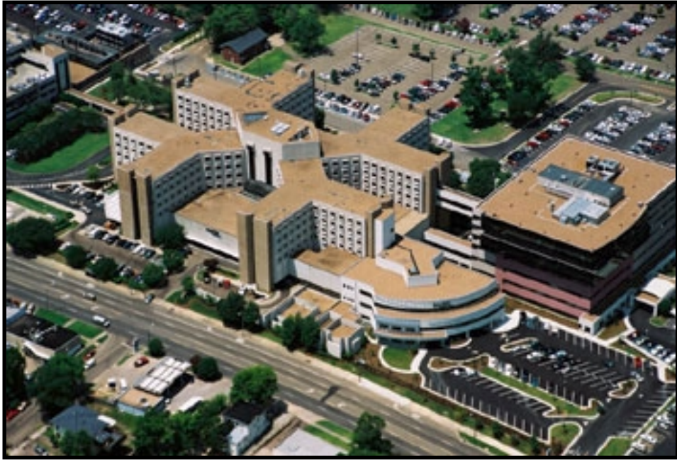
Figure 9.1: Site View of the MBMC
