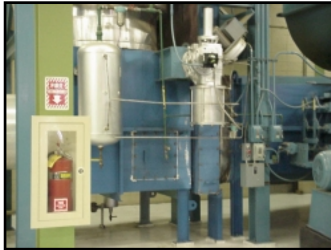
Figure. 9.4: Diverter Valve Arrangement
