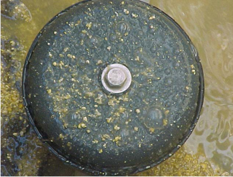
Figure 3.8. Ceramic diffuser used in the aeration system
