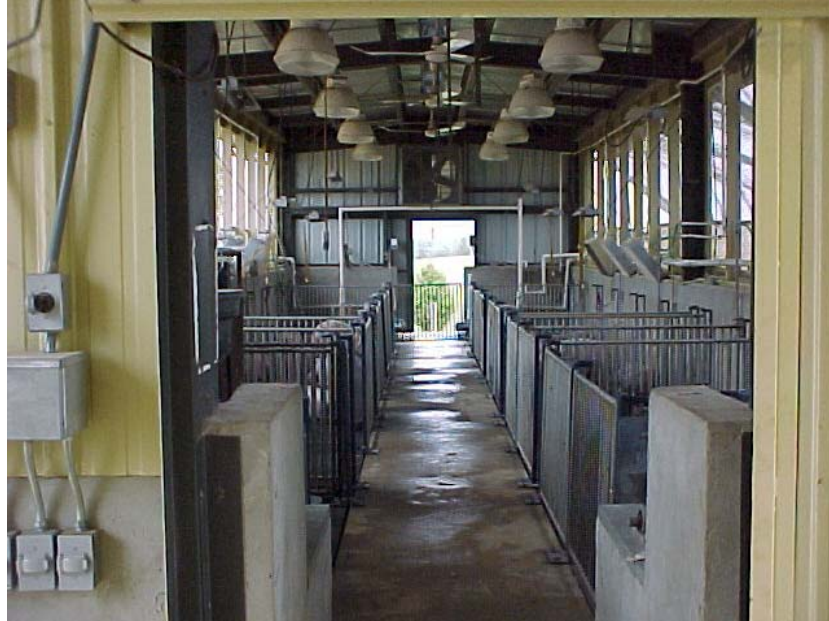
Figure 3.3. Inside view of barn
