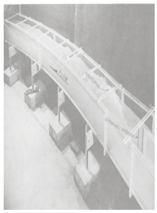
Figure 2.6: Standing Waves and Overtopping Downstream of Junction [Davis 87].
