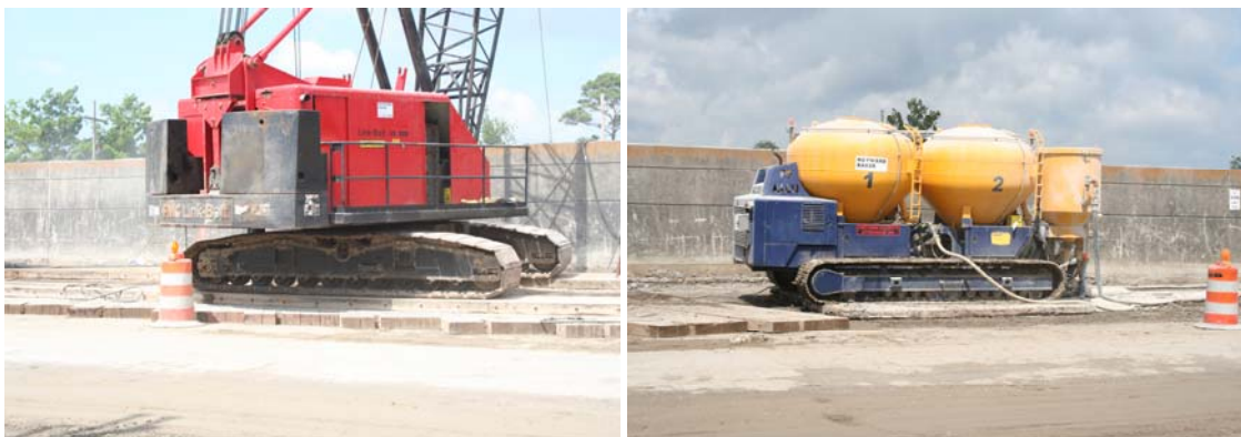
Figure 1.1 Wood Construction Platforms in Use
