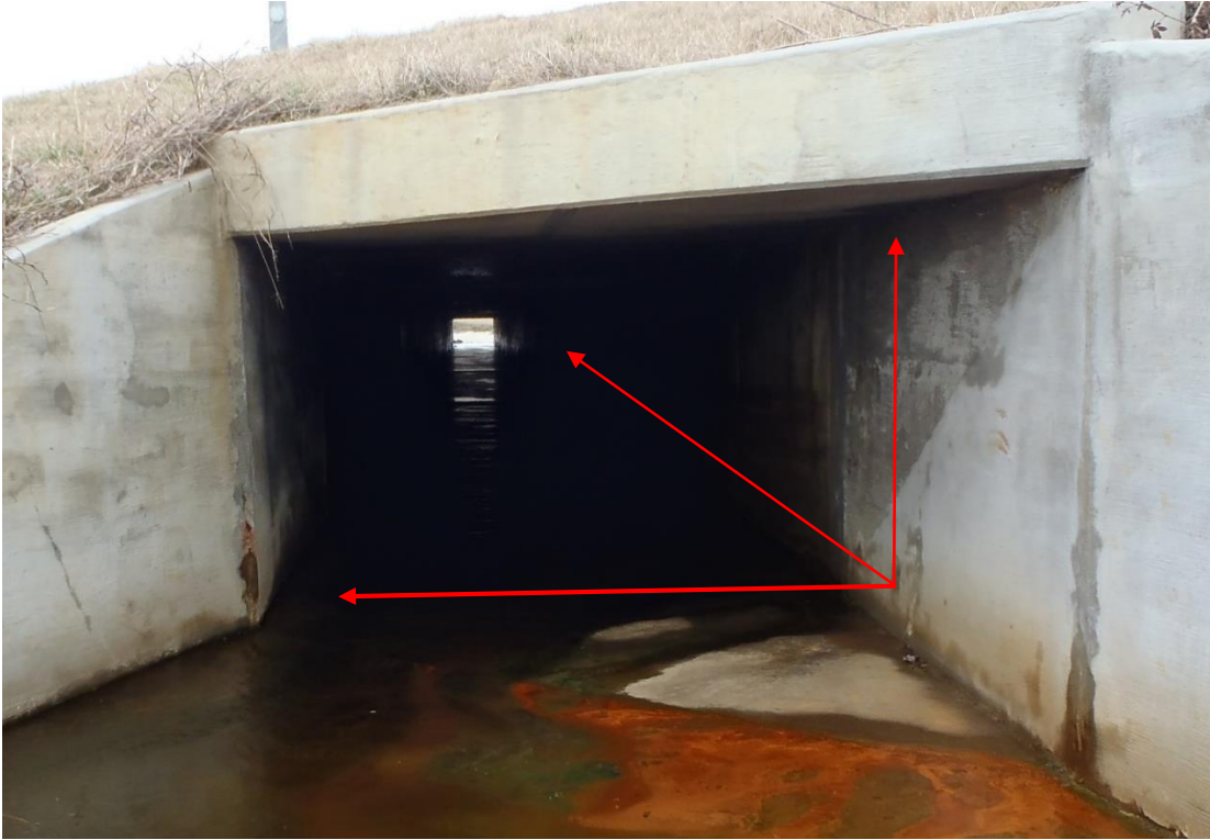
Figure 3.1 Measurement trajectories to estimate dimensions of culverts and box bridges in Mississippi study to estimate numbers and species of winter-roosting bats from 2010 through 2015.
