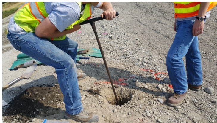
Figure 3.5 Hand Drilling of Instrumentation Holes.
