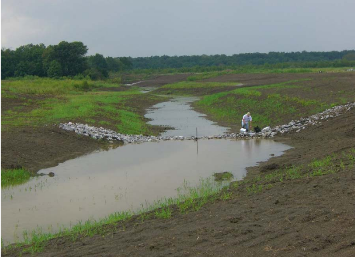
Figure 4.2 Terrace Ditch, Yazoo County, MS, immediately after implementation of weirs (September, 2009).
