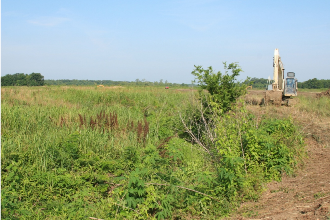
Figure 4.4 Terrace Ditch, Yazoo County, MS, prior to construction in 2009.
