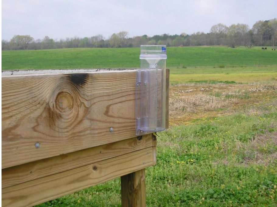
Figure 3.11 On-site rain gauge attached to roof platform.
