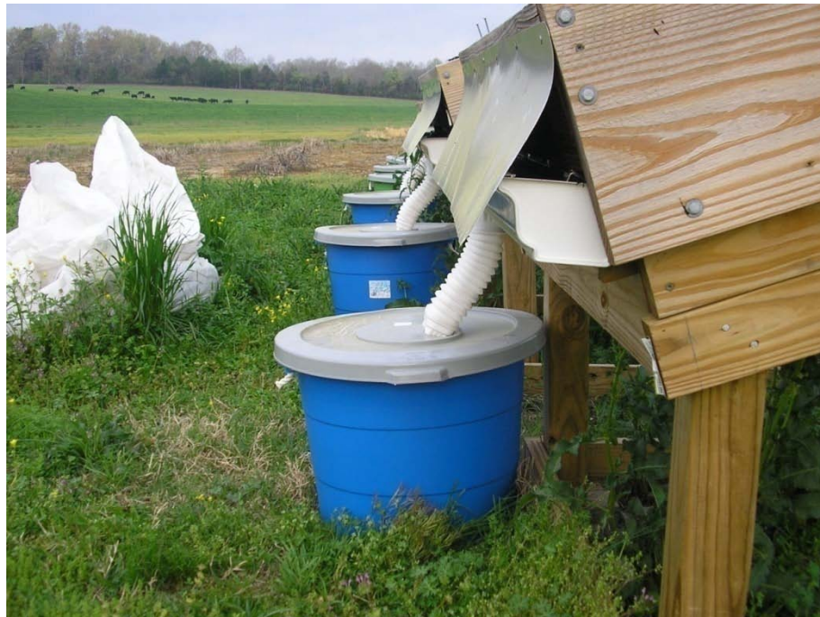
Figure 3.10 Stormwater runoff collection system.
