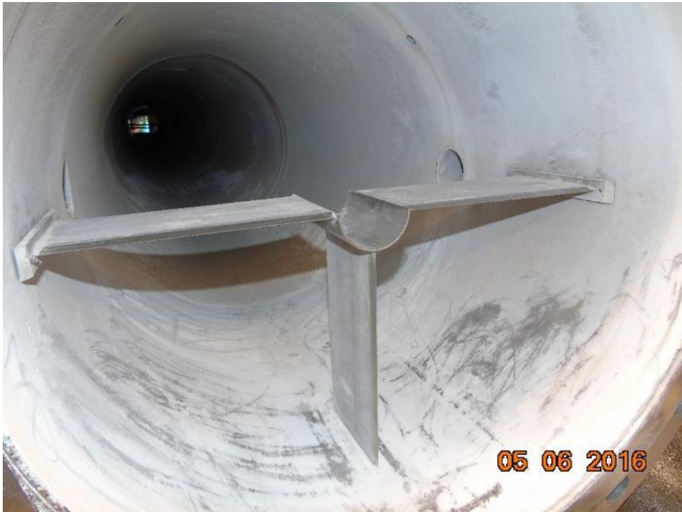
Figure 3.7 Pilat impactor cradle installed within the upstream ductwork.
