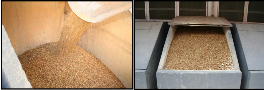
c) Aggregate Deposited into Bins
