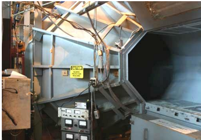
Figure 2.1 Previous Test-Section Configuration With Door Open
