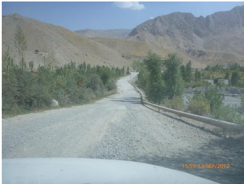
Figure C.20 Category 3 Classification 3 – Intermittent Gravel and Broken Pavement
