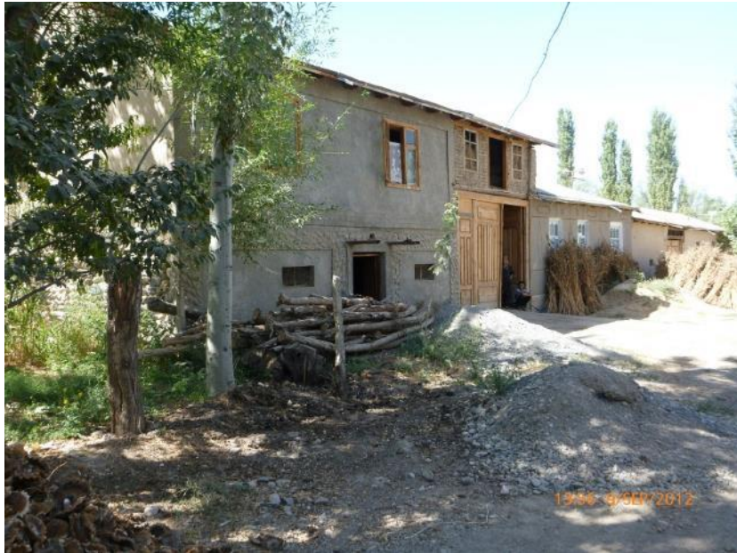
Figure C.31 External view of house built to high standards in Navobod
