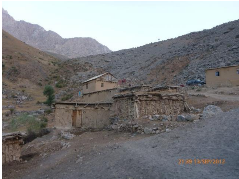
Figure C.38 7-Lakes District housing
