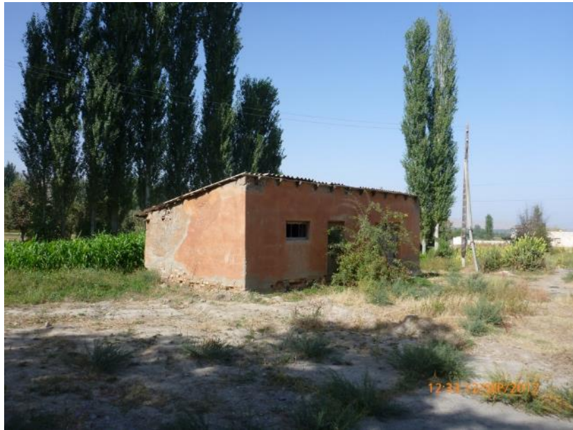
Figure C.12 Building housing primary school heating system, in disrepair
