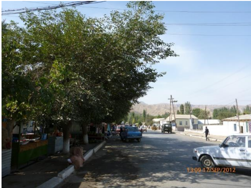
Figure C.18 Category 3 Classification 1 – Broken Pavement
