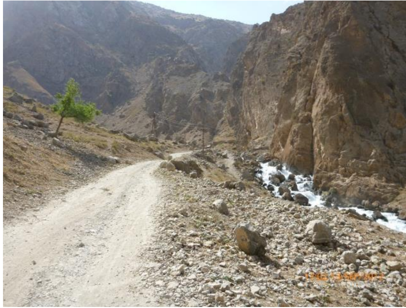
Figure C.21 Category 4 – 1-Lane Road; Travel frequency greatly reduced from Category 3
