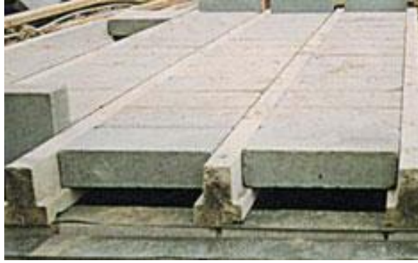
Figure 2.14 T-beam flooring
