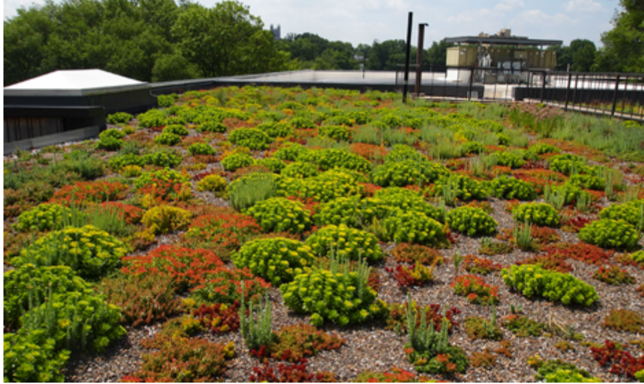
Sidwell Friends School Green Roof
