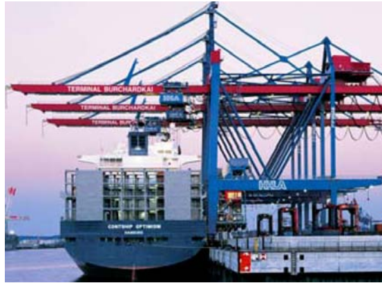
Figure 4 Quay Crane (Dual-Trolley)
