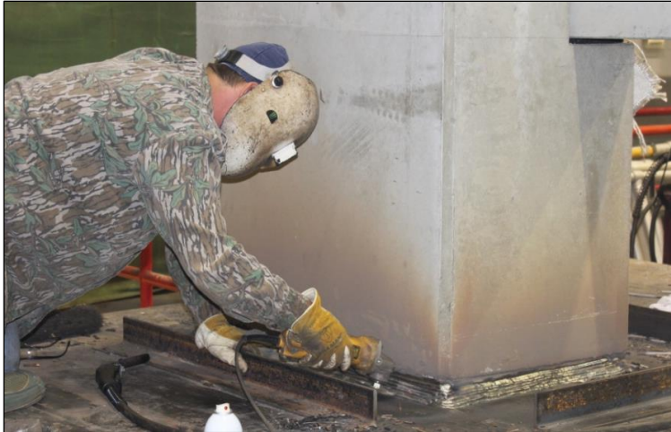
Figure 3.5 Welding of end-columns to reaction structure's footing
