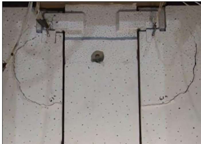
Figure 4.2 Elevation view, development of the first observed cracks in the beams near the top of the center column/stud, at \Delta of 0.38 in. (9.6 mm)
