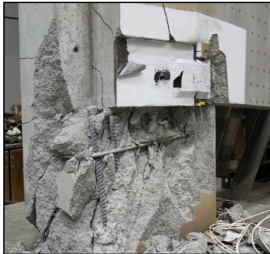
Figure 4.7 Elevation view, posttest damage of bottom of left (east) end-column
