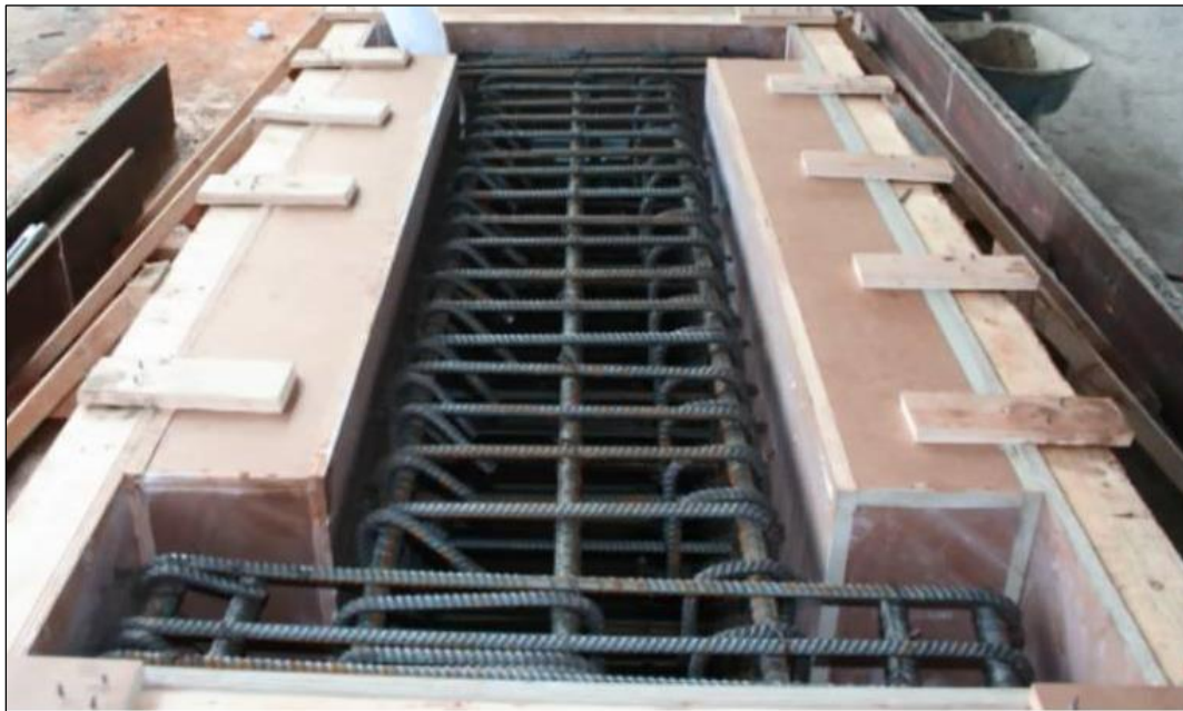
Figure 3.4 Concrete placement in OMRF's center column/stud
