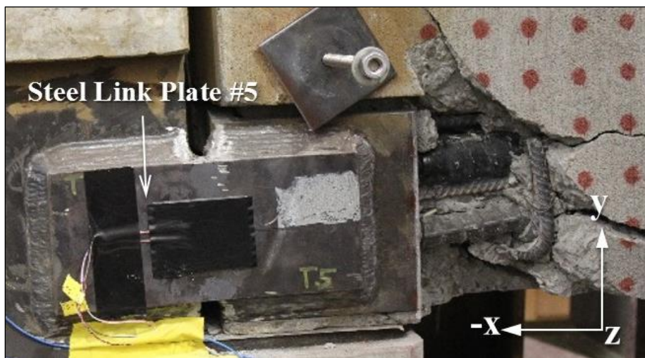
Figure 5.29 Close-up view to posttest damage steel link plate #5
