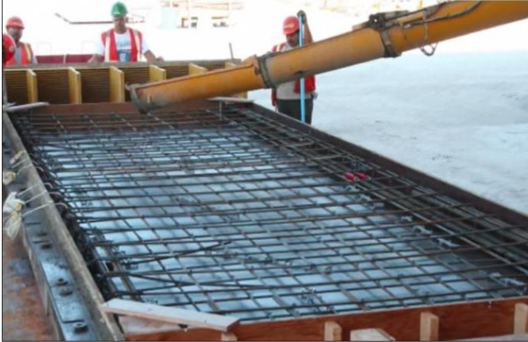
Figure 3.3 Concrete placement in OMRF's spandrel beam
