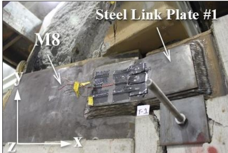
Figure 5.25 Close up view to posttest damage steel link plate #1
