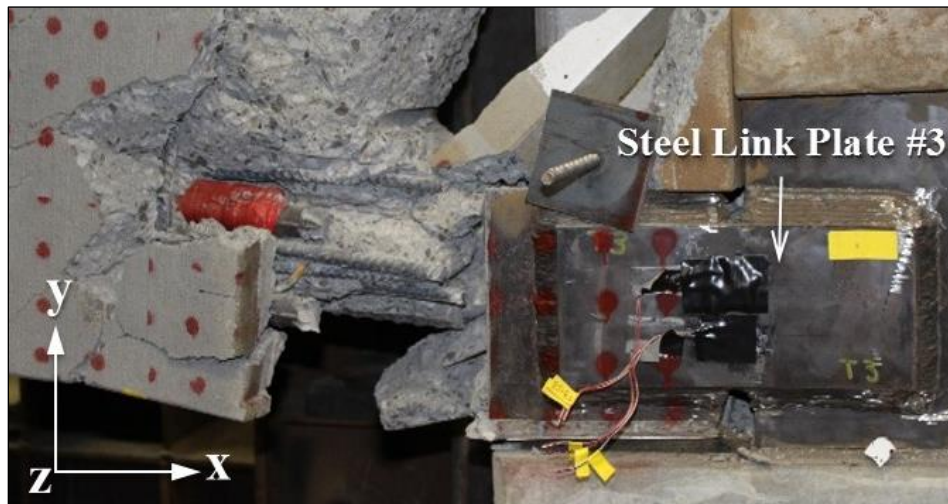
Figure 5.27 Close up view to posttest damage steel link plate #3
