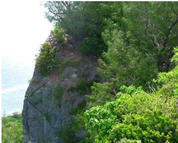
Figure 43 Low angle joints that may cause cliff edge rock collapses.
