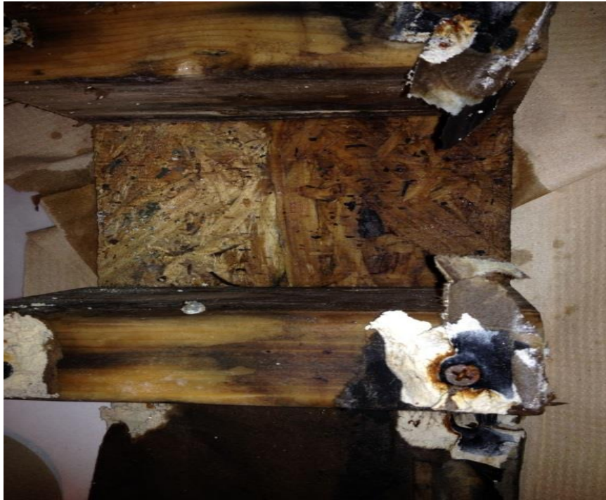
Figure 3.9 Picture of dismantled wall on day 65.
