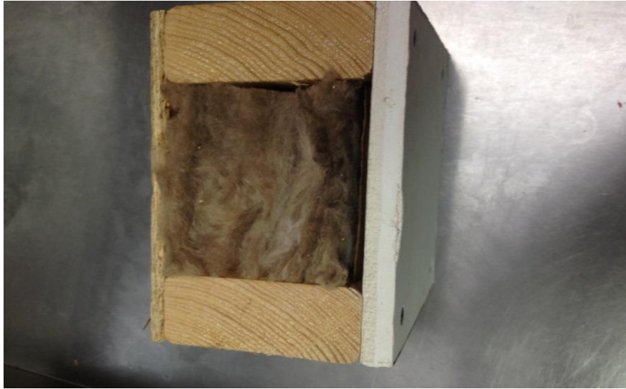
Figure 2.5 Picture of the inside of the residential building wall showing the wood studs and batt insulation.
