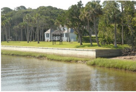
Kingsley Plantation main house
