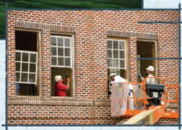
Crews focus efforts on restoration work for the Lloyd-Ricks building.
