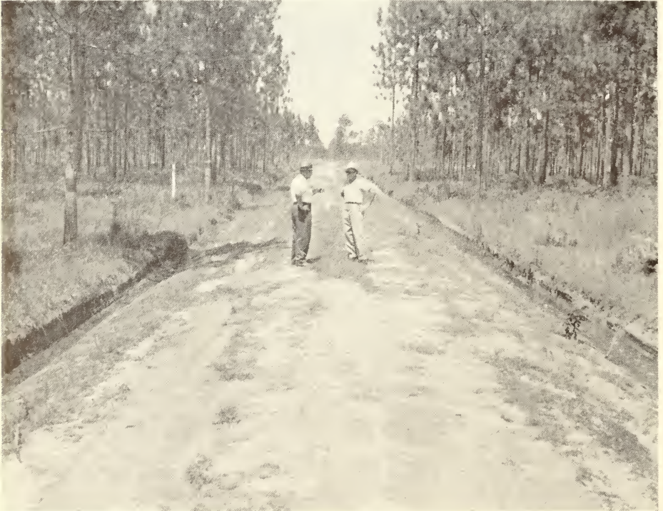
This road serves as an access road, a drainageway, and a fire break. (Courtesy of Soil Conservation Service)
