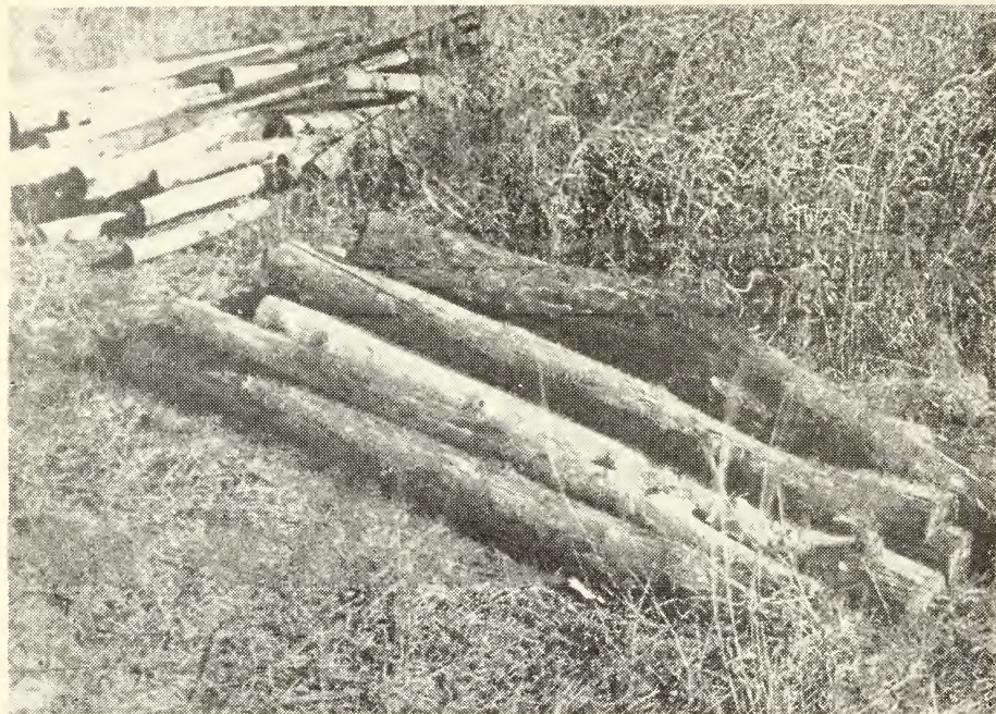
Figure 4. Very poor piling practice.
