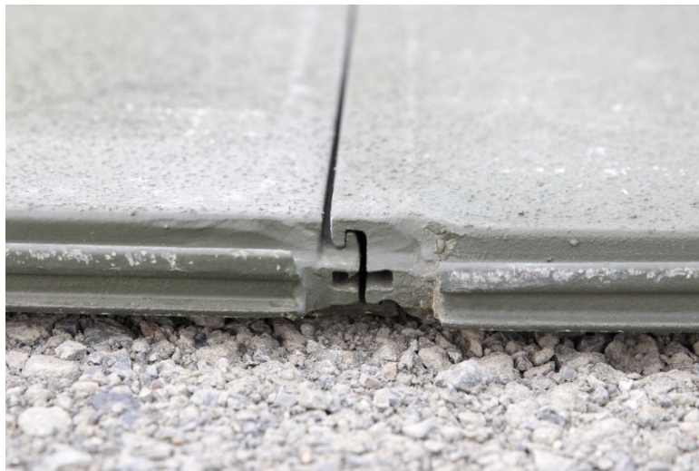
Figure 2 Photograph of the AM2 locking connection
