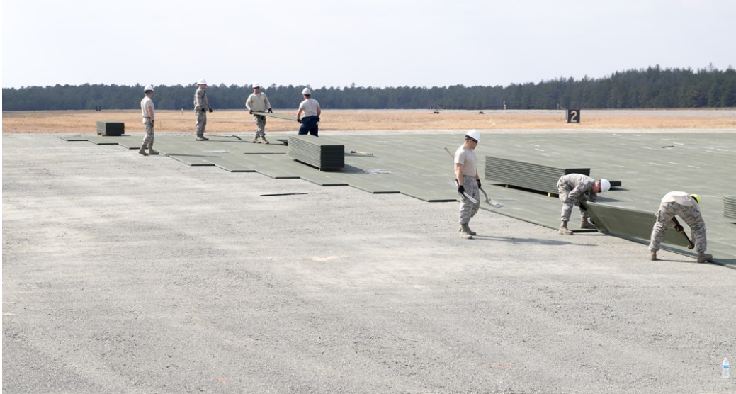
Figure 1 Photograph of AM2 matting installation
