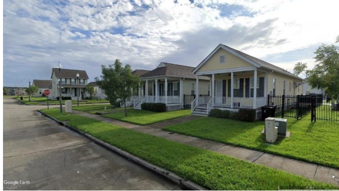
Figure 4.31 The Fischer Site Representative Cottage in New Orleans, Louisiana
