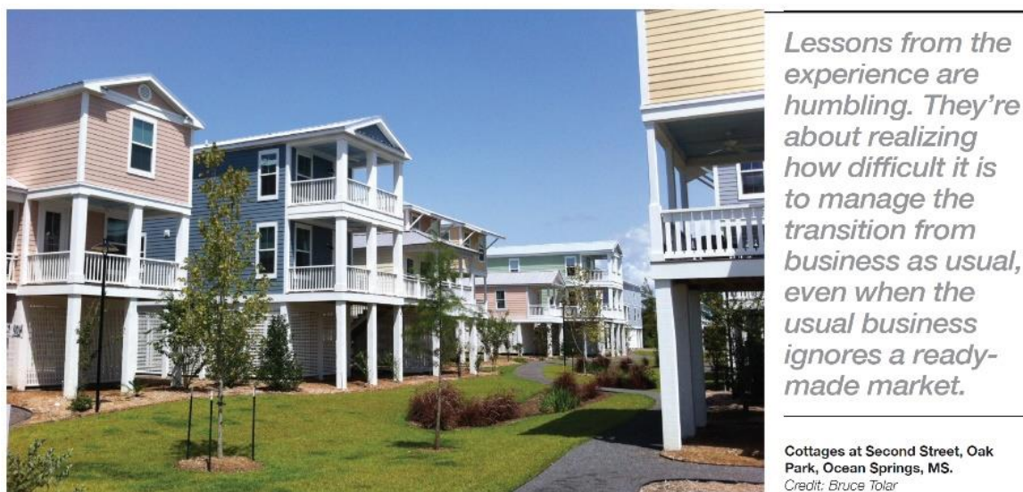
Figure 2.23 Photos of the Cottages at Second Street in Pass Christian, Mississippi (Tolar & Brown, 2015, p. 4)
