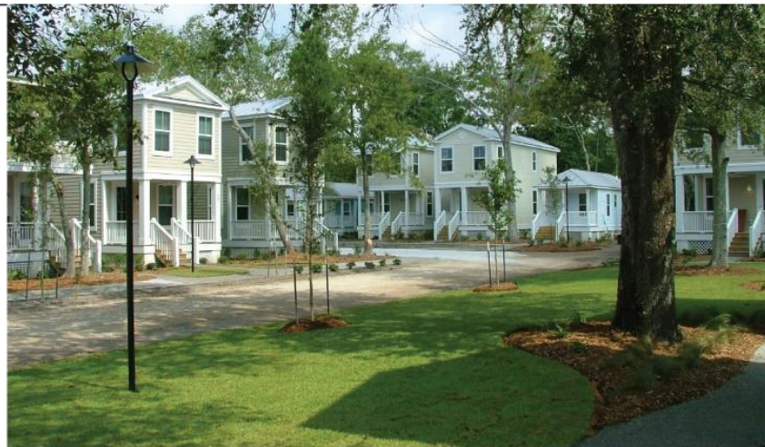
Figure 2.22 Photos of the Cottages at Oak Park in Ocean Springs, Mississippi (Tolar & Brown, 2015, p. 3)
