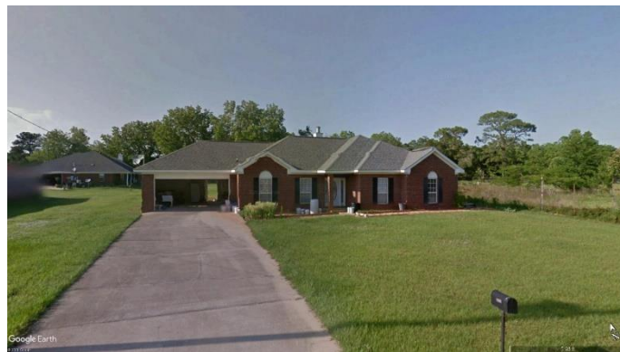
Figure 4.51 Small Single-Family Home Comp in Bayou La Batre, Alabama
