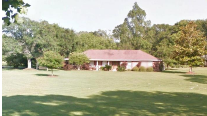
Figure 4.52 Large Single-Family Home Comp in Bayou La Batre, Alabama
