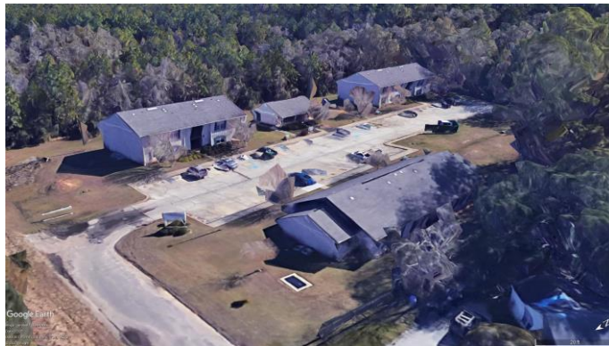
Figure 4.53 Apartment Comp in Bayou La Batre, Alabama
