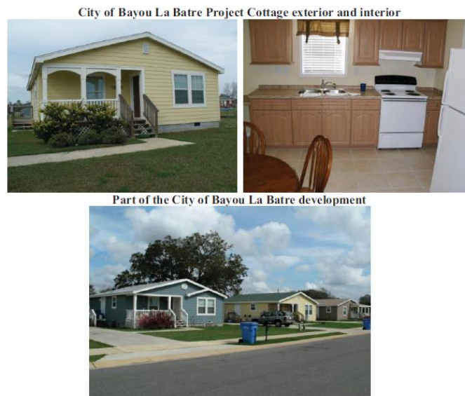
Figure 2.28 Katrina Cottages at Safe Harbor
