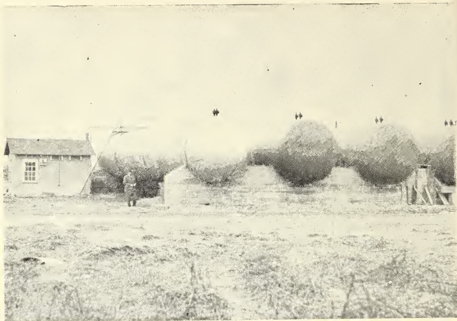
Figure 6. A bulk storage plant consisting of four 30,000-gallon high pressure tanks. The compressor for loading and unloading is located in the small house.
