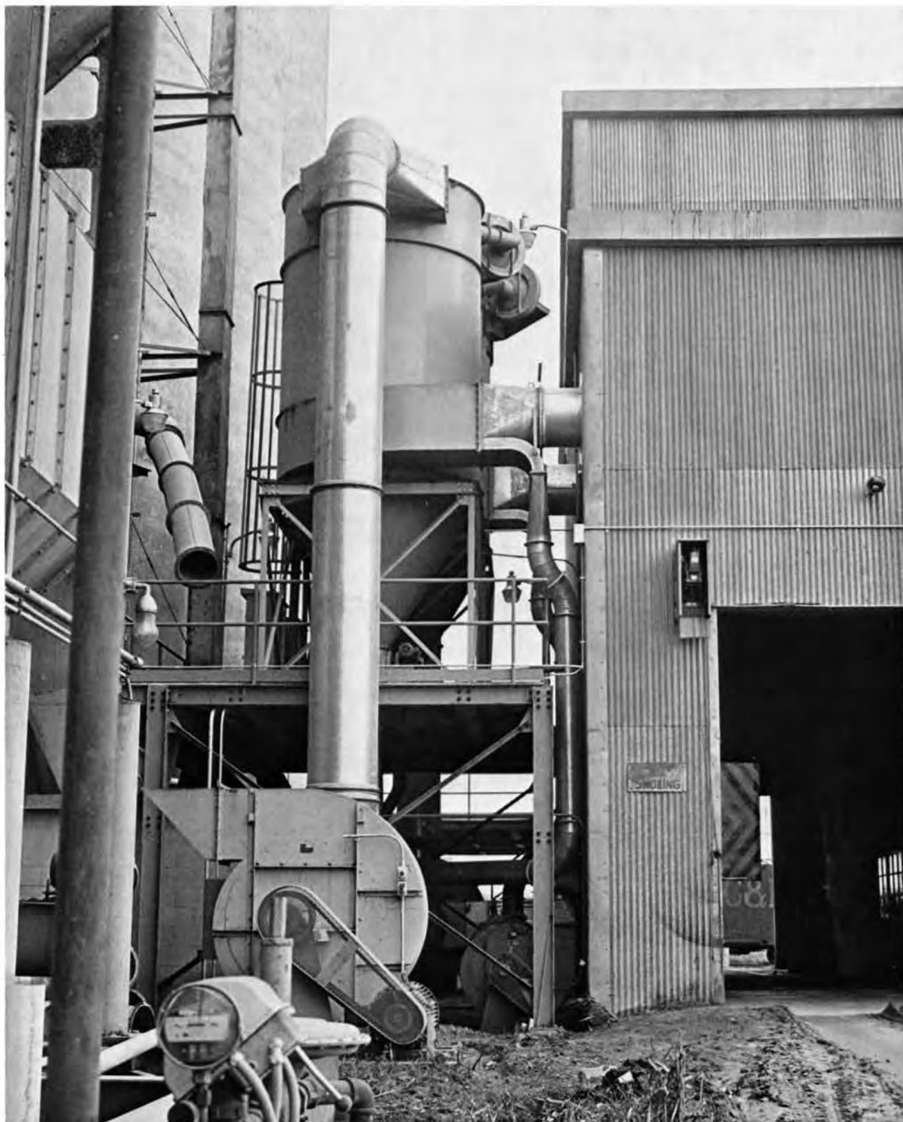
Figure 9. Typical RJ dust filter installation.
