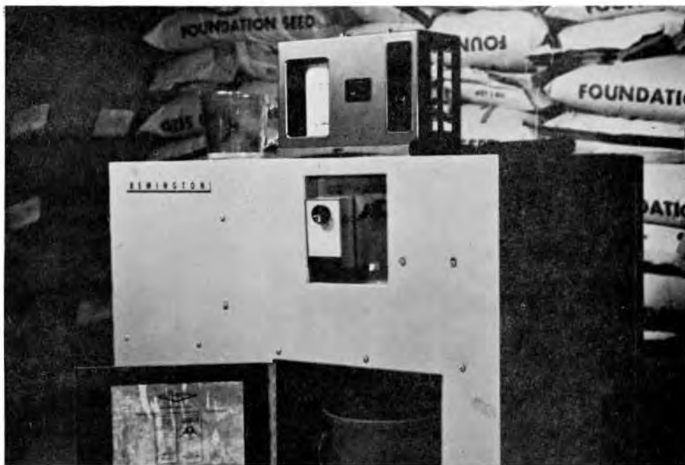
Figure 6. A refrigeration type dehumidifier located inside a seed storage room. Moisture is condensed out of the air and collected in a bucket or piped out of the room.
