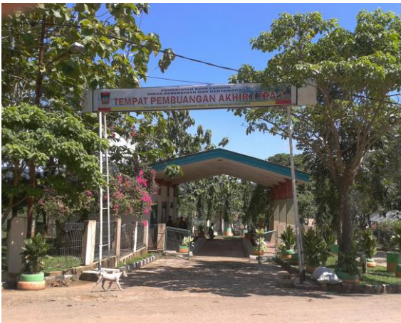
Figure 1. Main Gate of TPA Air Dingin
