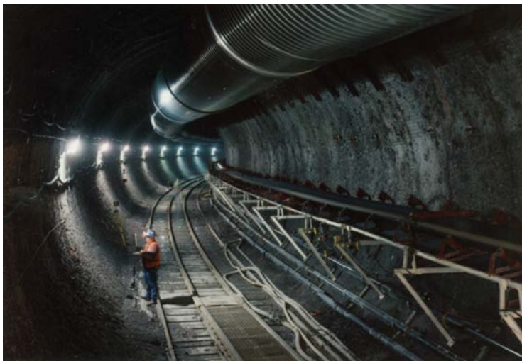
Fig 2. First curve of the main tunnel of the exploratory studies facility at Yucca Mountain, Nevada, October 1995. (US DOE, http://energy.gov/photos/yucca-mountain ).
