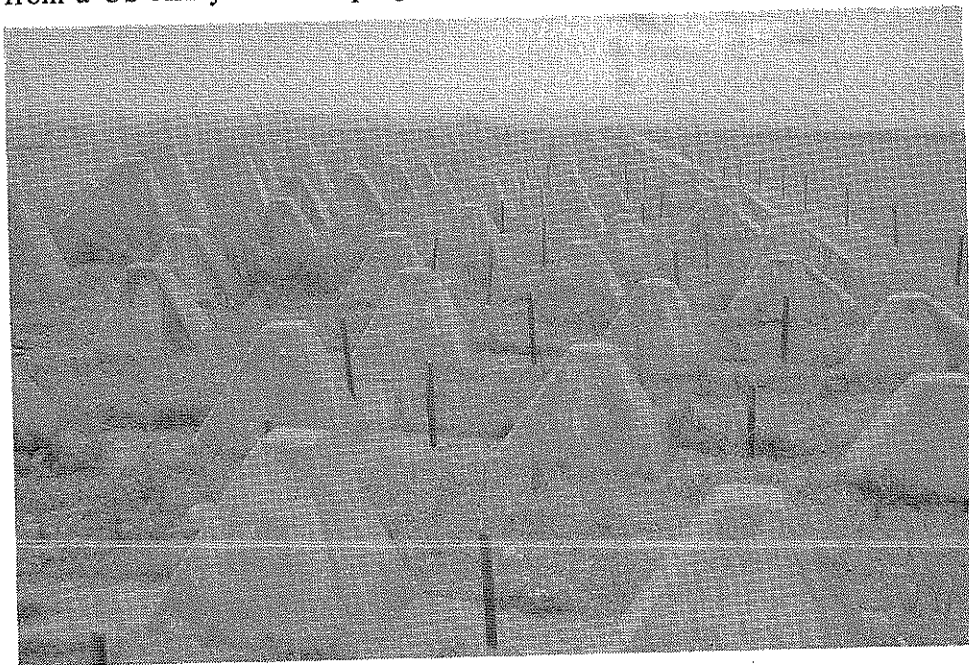
Too obtrusive to construct in West Germany today, but an effective wartime obstacle fifty years ago, these concrete dragon's teeth formed part of the Siegfried Line. This photo was taken near Lammersdorf, Germany, on 25 September 1944.
