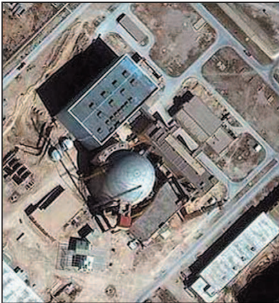
Figure 1. Bushehr Light Water Reactor.
