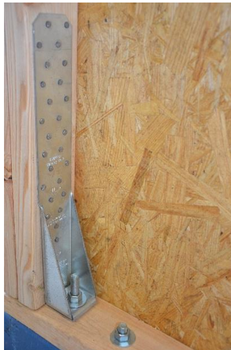
Figure 4. Simpson HTT5 Hold-Down
