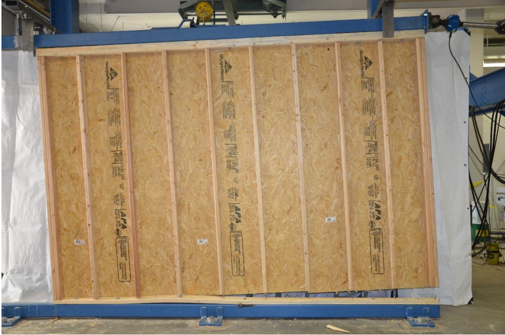
Figure 20. Stud pullout from bottom sill plate failure mode
