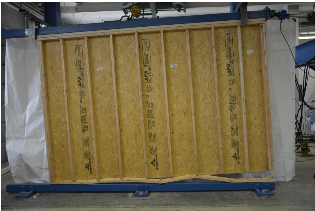
Figure 21. Bottom sill plate splitting failure mode
