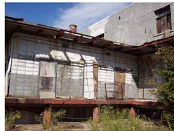
Figure 70. CMU Addition Author
