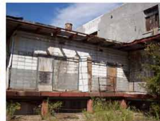
VIEW TOWARDS ONE STORY CMU ADDITION
