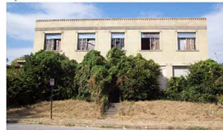
Figure 71. Existing South Facade Author
