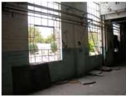
VIEW OF EXISTING WINDOWS
