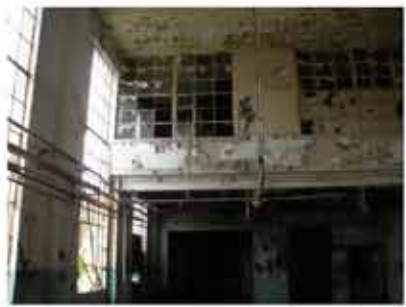
VIEW INSIDE DOUBLE-HEIGHT SPACE
