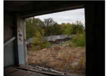
VIEW TOWARDS GREEN ROOF ON ADDITION
