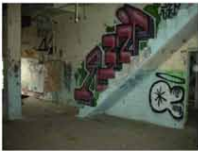
VIEW OF EXISTING STAIR
