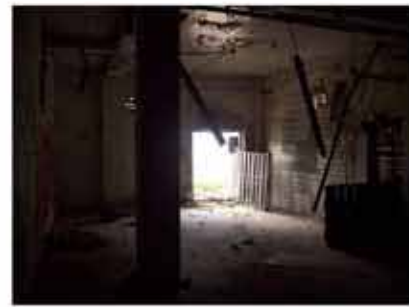
VIEW TOWARDS LOADING DOCK
