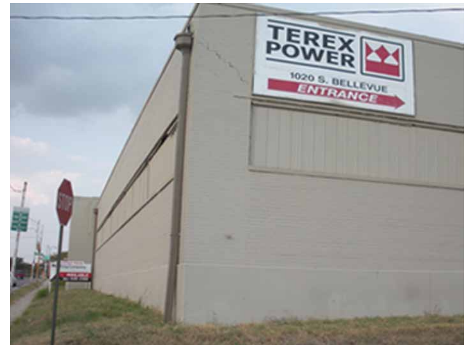
Figure 65. Terex Power Warehouse Author
