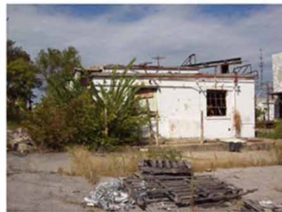
Figure 69. Additional Warehouse Author
