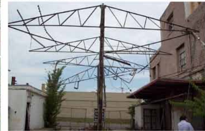
VIEW TOWARDS EXISTING METAL TRUSS STRUCTURE
