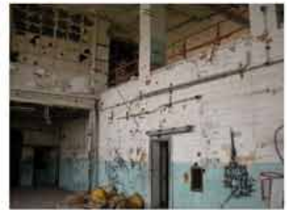
VIEW TOWARDS MEZZANINE
