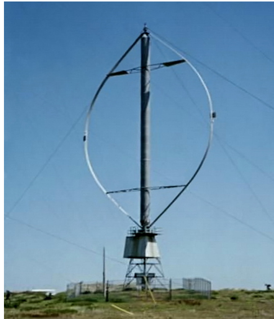
Figure 13. Vertical axis wind turbine [5]
