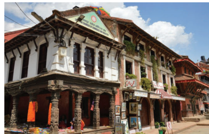
Pati incorporated at first floor of a community building
