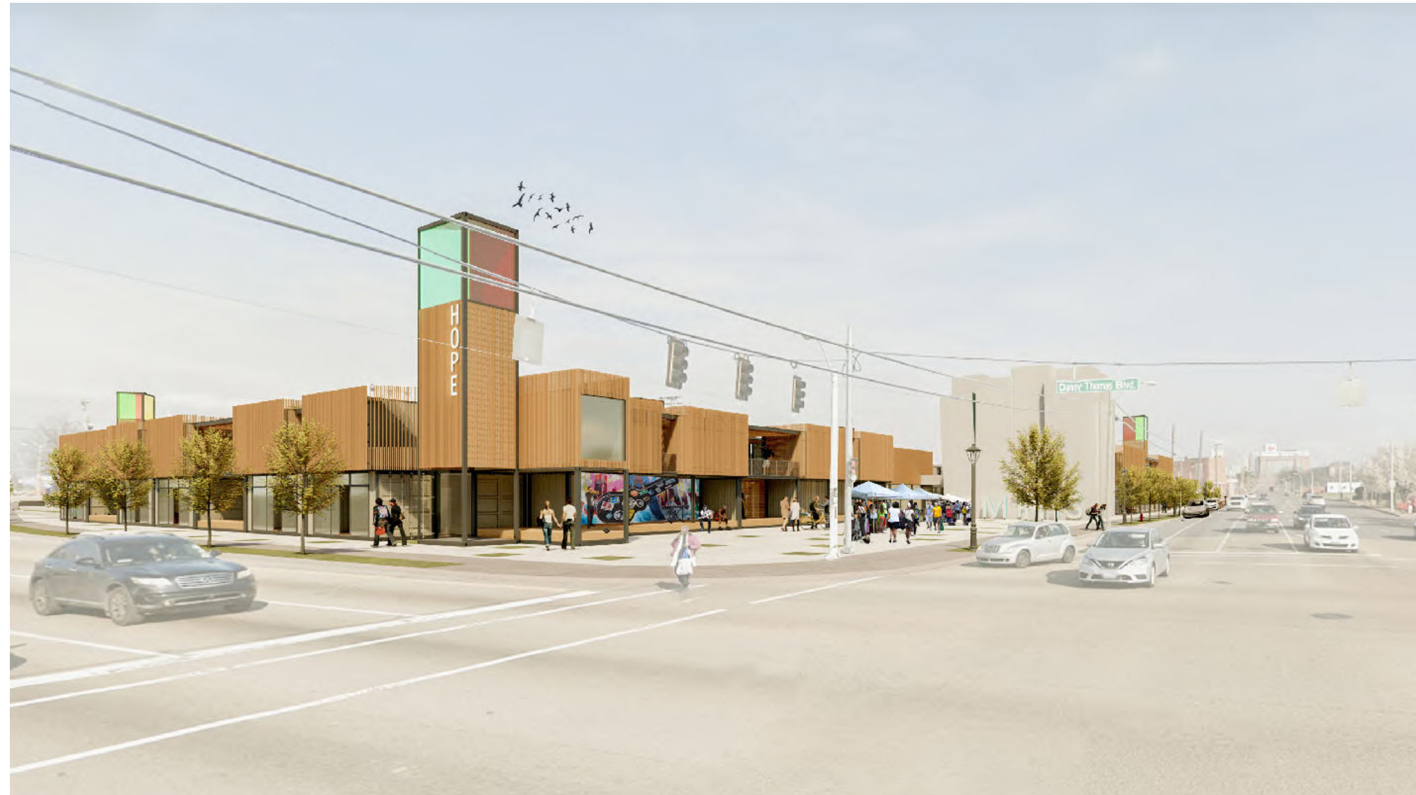
Figure 80 West Street Plaza
