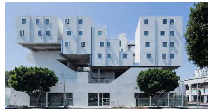
Building exterior with retail at base and residential module at top
