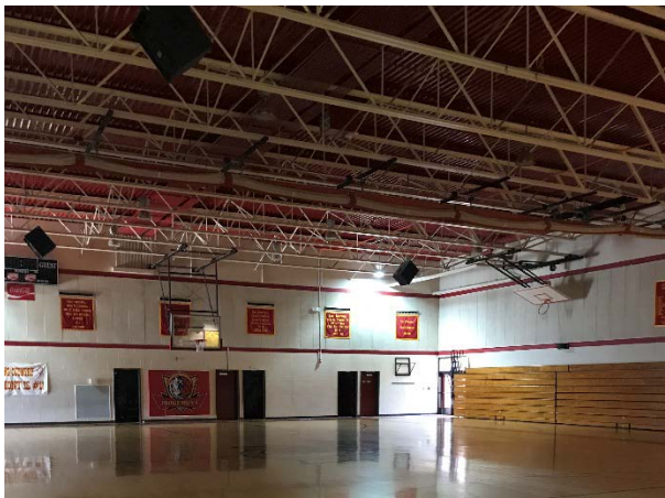
Flexible Diaphragm Roof
