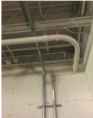
Interior, Reinforced Masonry, Flexible Roof System
