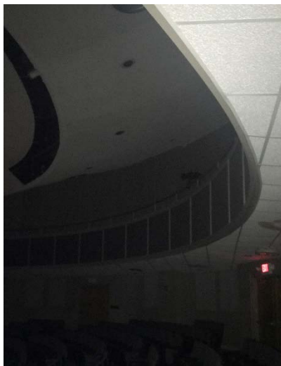
Interior, Split Level
