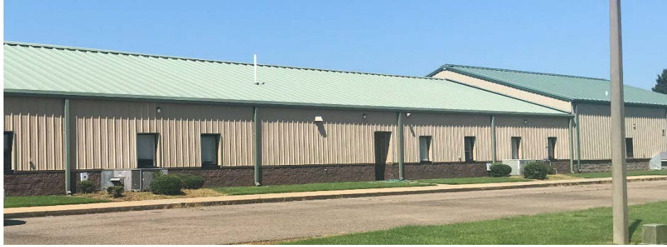
Structure 46 Lower Roof, Structure 47 Higher Roof
