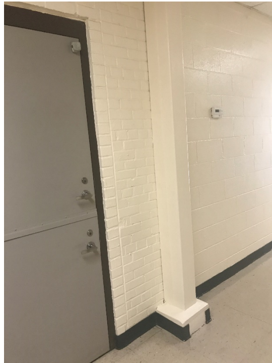
Interior, Joint between Structures 38 and 39
