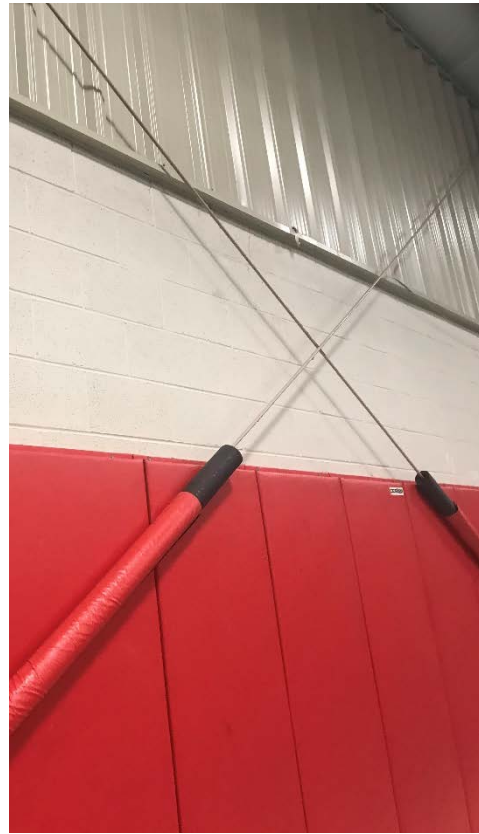
Interior, Exposed Wall
