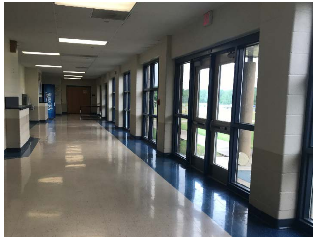
Interior, Masonry and Possibly Steel
