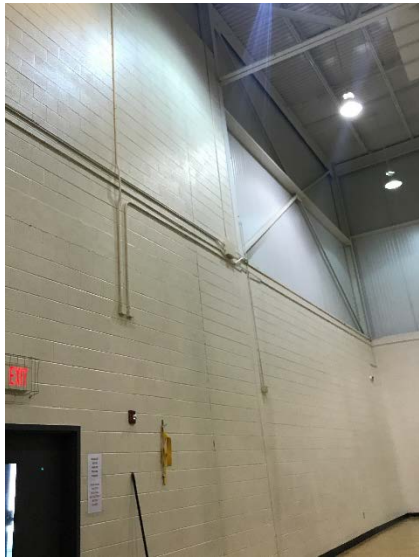
Interior, Steel Framing Exposed
