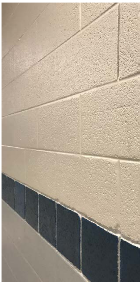
Interior, Reinforced Masonry
