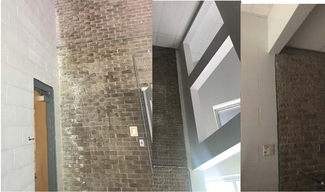
Joints Between Structure 58 and 59
