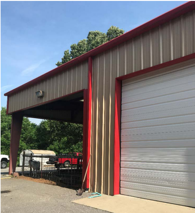
Exterior, Side of Building
