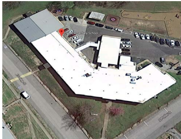
Plan View, Structure 40 is L-shape and Green Roof Portion Structure 41 has a Hallway and Breezeway Connection to Main Building
