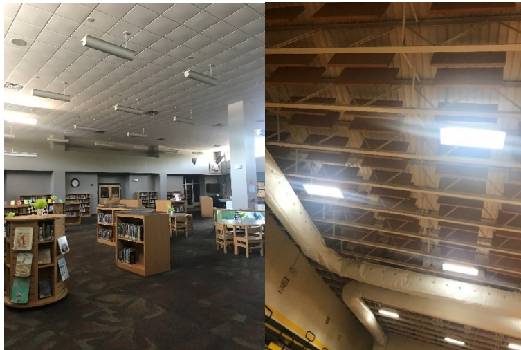
Previous Courtyards Filled-in to Build Library and Gym
