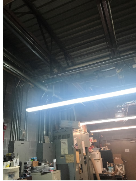
Interior, Mechanical Room, Exposed Ceiling and Walls
