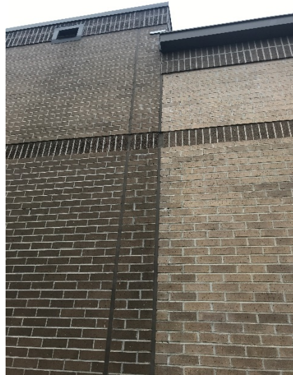
Joint between Structures 1 (Left) and 2 (Right)
