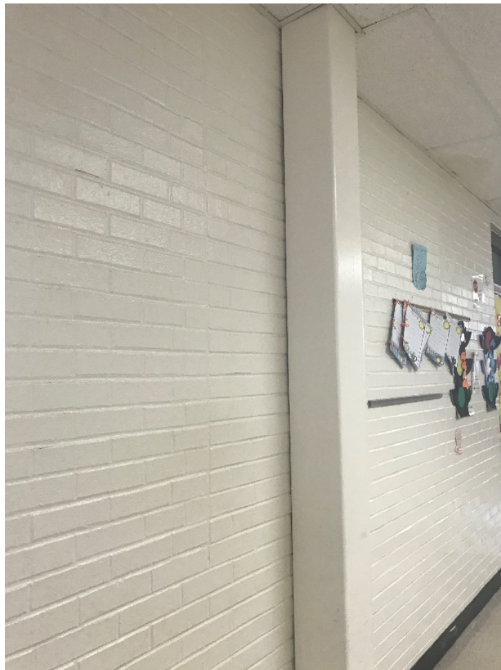
Previous Exterior of Structure 31, Column Added to Support Addition of Structure 32
