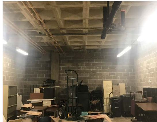
Interior, Exposed Concrete System
