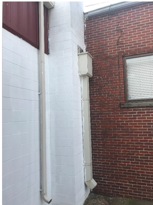
Exterior, Connection to Older Portion
