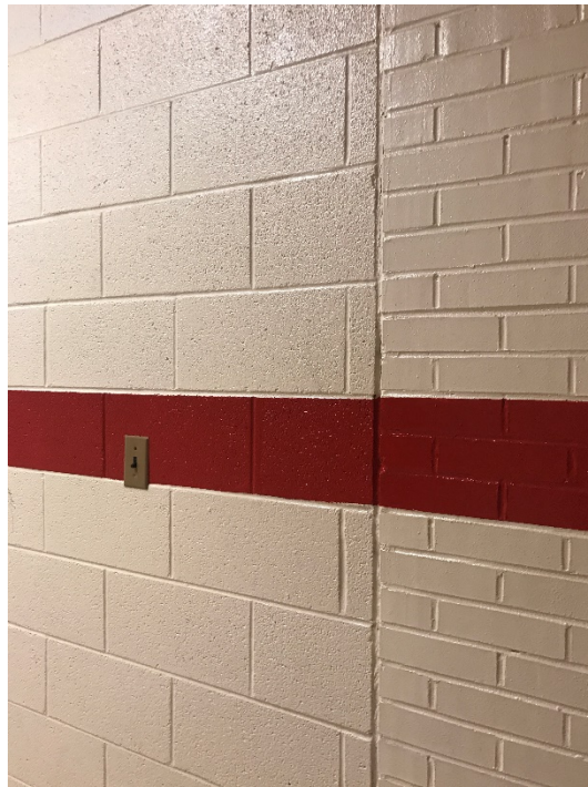
Interior, Connection to Addition
