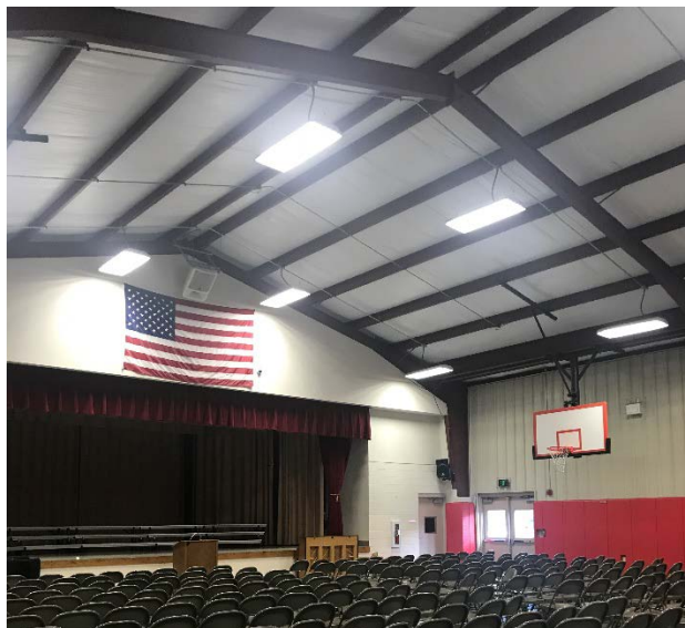
Interior Gym/Theater, Wall and Ceiling Exposed
