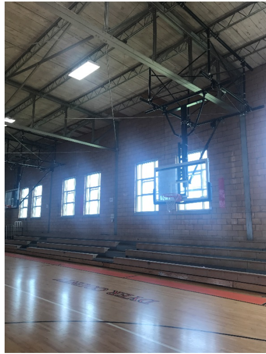
Interior, Masonry and Steel Exposed
