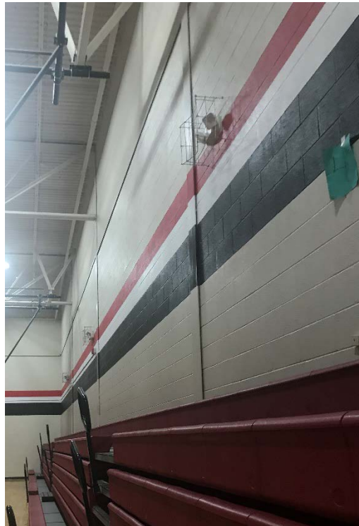
Steel Columns Exposed
