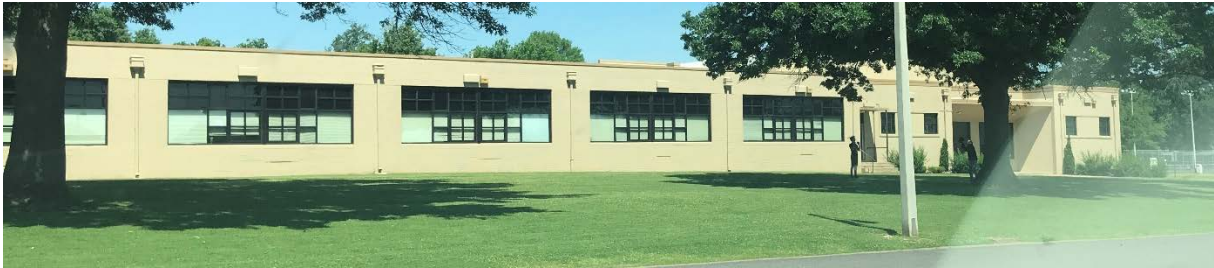
Front Right Exterior, Primary Hallway That Wings Come From, All Sides Similar
