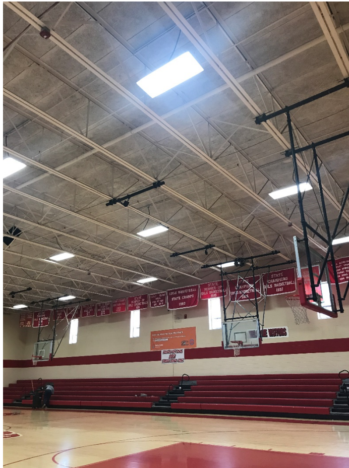
Interior, Gymnasium, Walls and Ceiling Exposed
