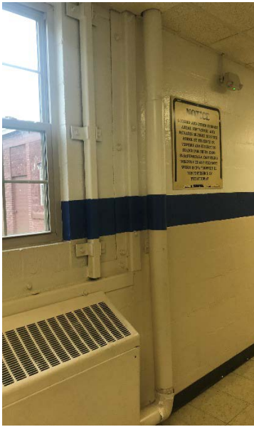
Added Reinforcement (1 of 2)
