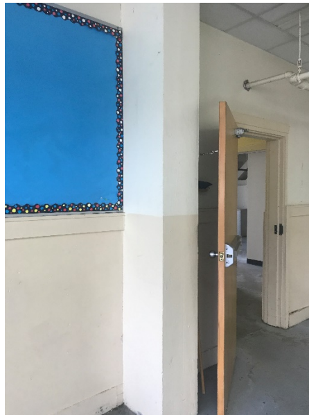
Interior, Concrete Pillars in Half-Basement Level
