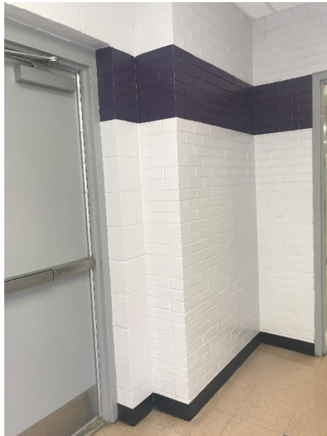
Joint Between Structures 84 (Right) and 85 (Left)
