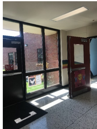
Connection from Structure 49 to 50
