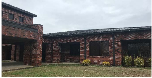
Exterior of Structure
