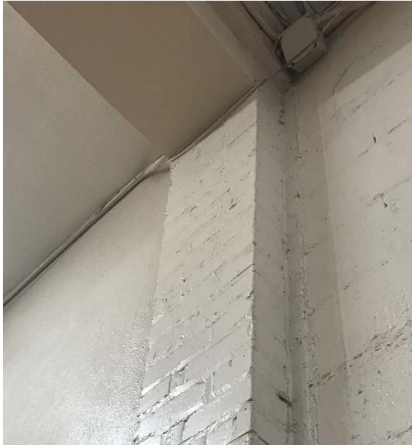
Interior, Encased Steel Column
