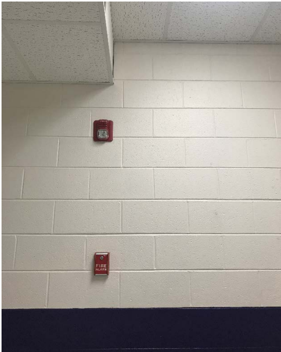
Interior, Masonry Walls
