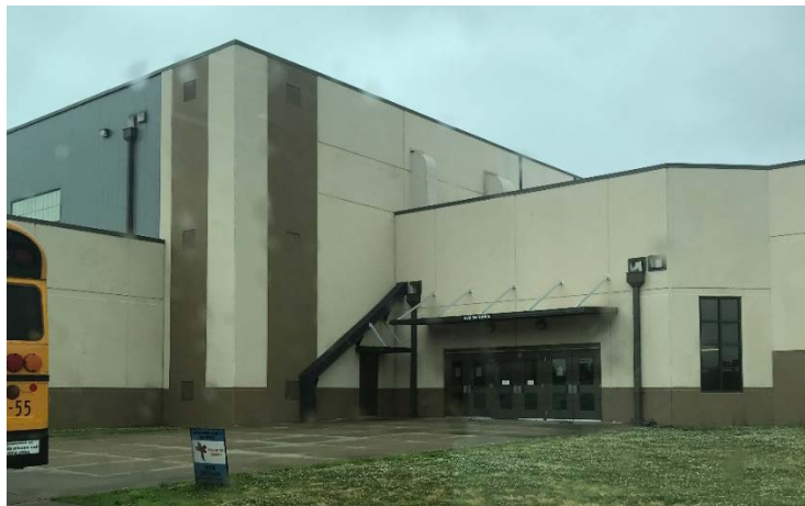
Exterior, Split Level, Out-of-Plane Setback
