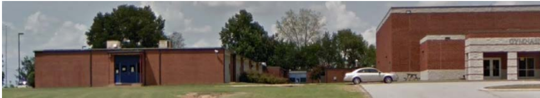
Left is Structure 79, Right is Structure 80, Connected by Hallway
