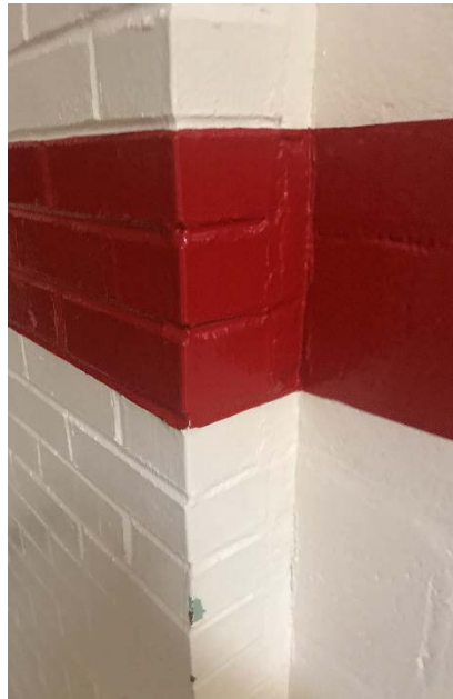
Interior, Connection Between This Structure and Addition
