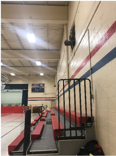
Gymnasium, Exposed Roof
