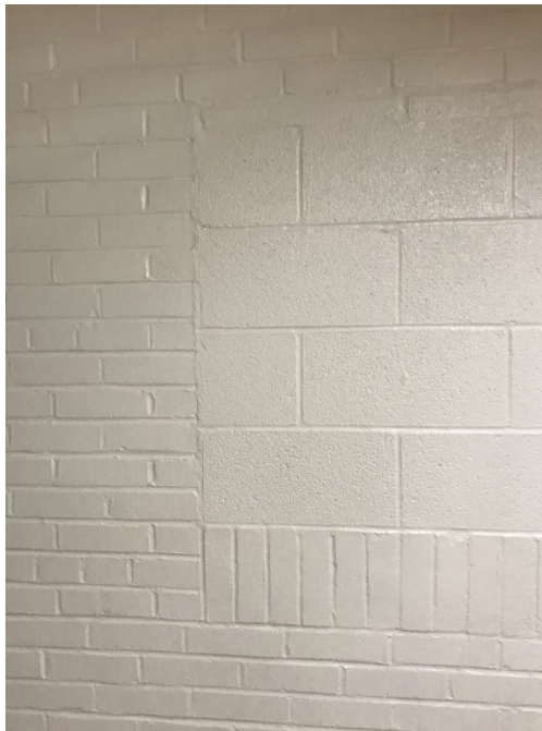
Updated Section (Covered Older Large Window Opening)
