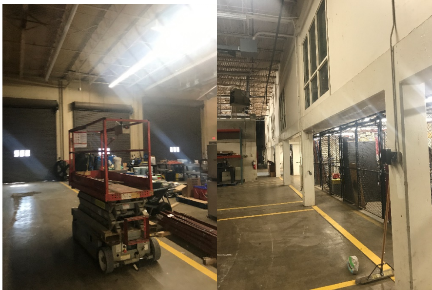
Interior, Split Level, Concrete Columns Exposed
