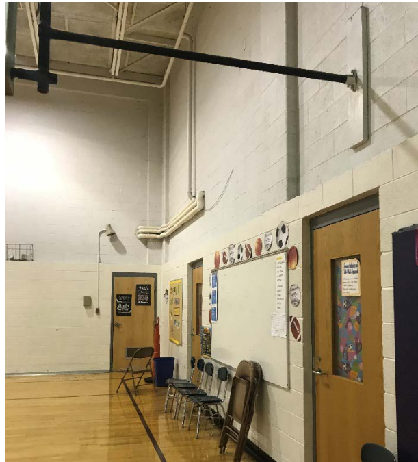
Interior, Gymnasium, Exposed Walls and Ceiling
