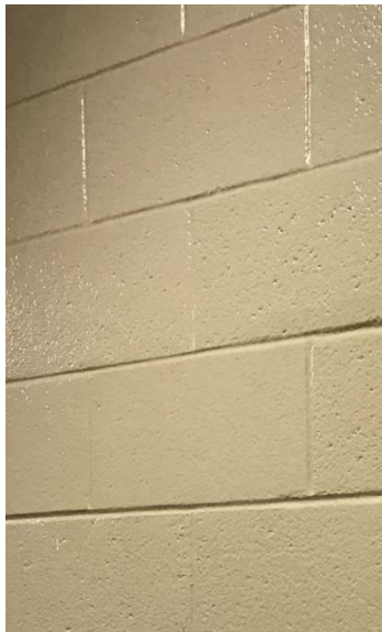
Interior, Reinforced Masonry
