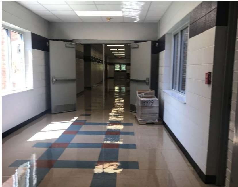
Structure 85 is One Hallway Addition to Structure 84
