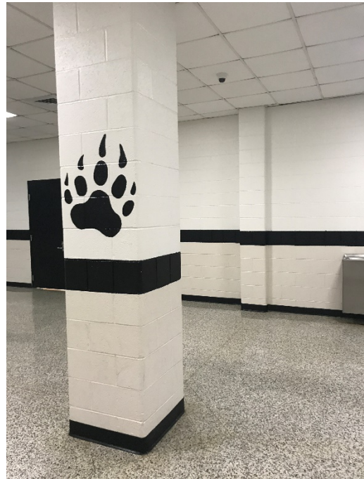
Interior of Structure
