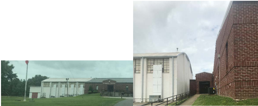
Exterior, Joint between Structures 31 and 32
