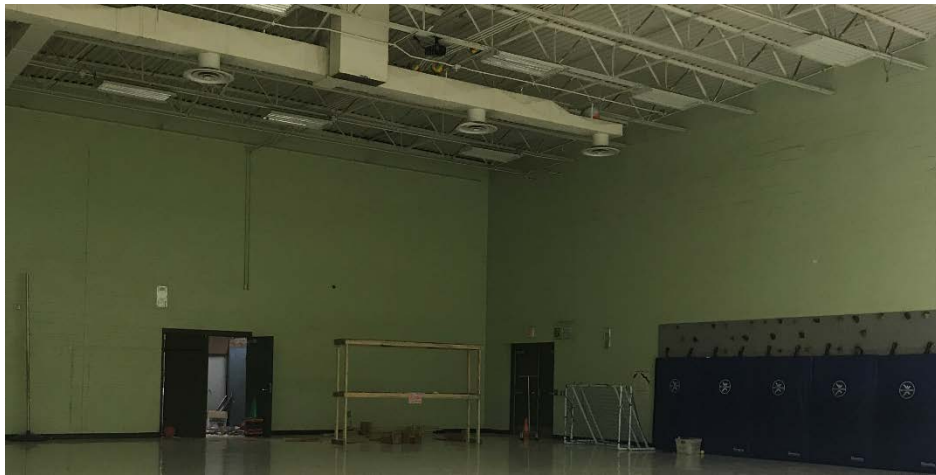
Interior, Gymnasium, Flexible Diaphragm Roof
