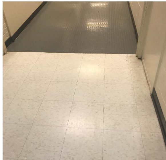
Connection to New Hallway to Newer Building
