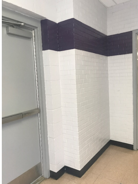
Joint Between Structures 84 (Right) and 85 (Left)
