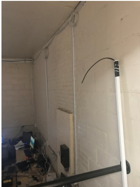
Interior, Openings Filled in with Bricks
