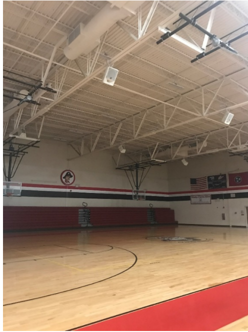
Gymnasium, Steel Truss System at Roof
