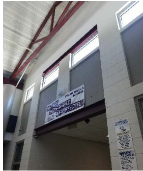
Interior, Split Level
