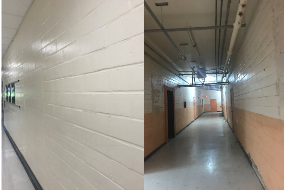
Interior, Aged Masonry
