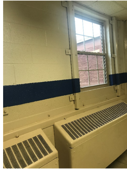
Added Reinforcement (2 of 2)
