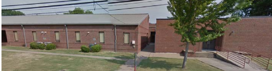
Exterior, Structure 38 Right and 39 Left
