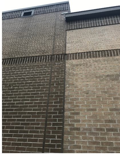
Joint between Structures 1 (Left) and 2 (Right)
