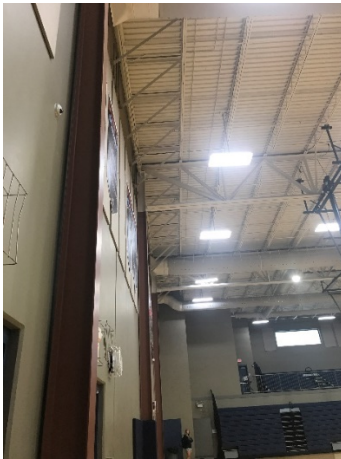
Interior, Exposed Ceiling in Gymnasium
