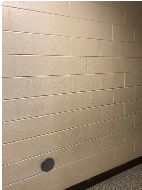
Interior, Reinforced Masonry
