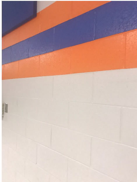
Interior, Reinforced Masonry
