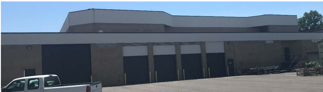
Exterior, Out-of-Plane Setback
