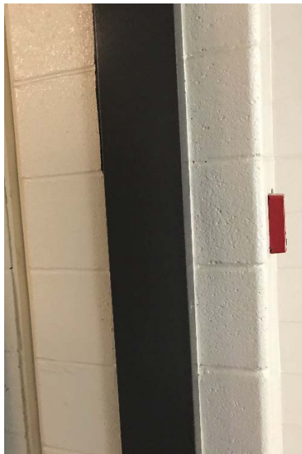
Firewall Between Structures 70 and 71
