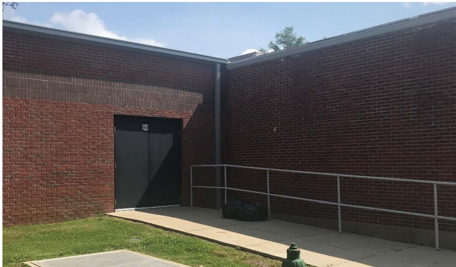
Exterior of Addition
