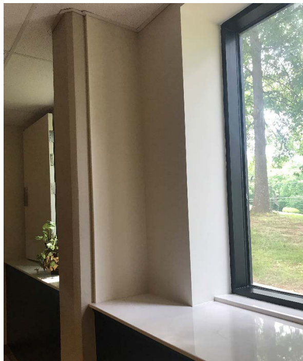
12" Thick Concrete Walls and Exposed Concrete Columns, Safety Windows
