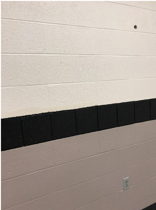
Interior of Structure
