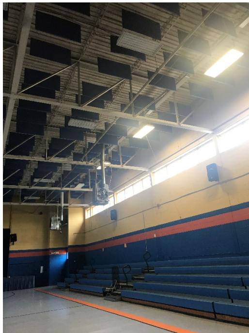
Steel Columns in Gym
