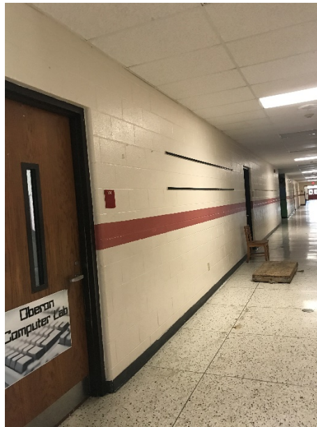
Interior, Reinforced Masonry
