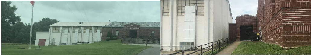
Exterior, Joint between Structures 31 and 32
