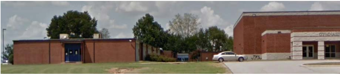
Left is Structure 79, Right is Structure 80, Connected by Hallway
