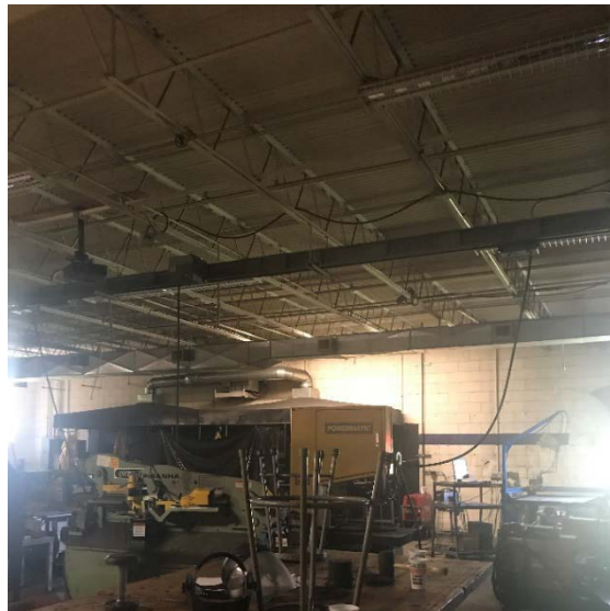
Interior, Flexible Roof System
