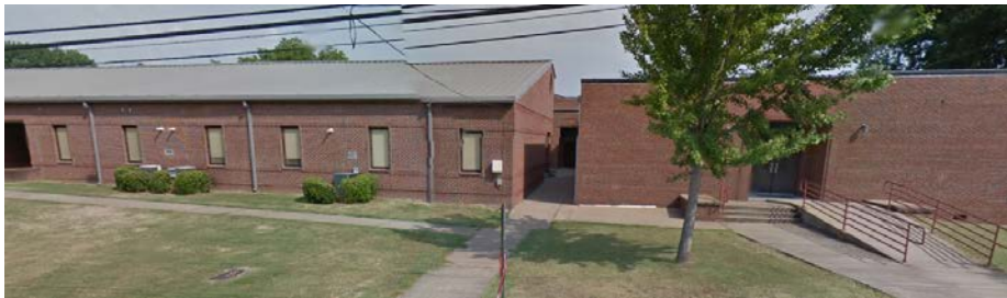
Exterior, Structure 38 Right and 39 Left
