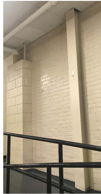
Interior, Exposed Steel Column
