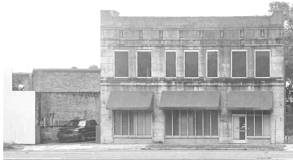
Figure 16 The Edge District, Front Facade of Masonry Building
