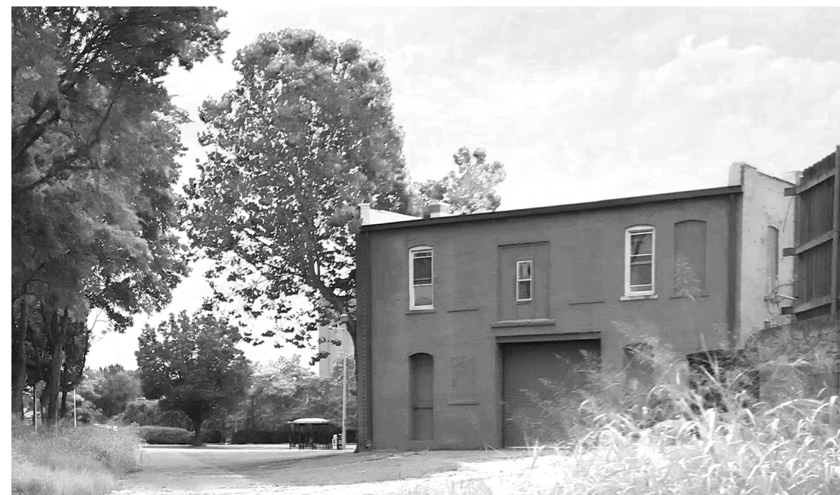
Figure 17 The Edge District, Rear Facade of Masonry Building
