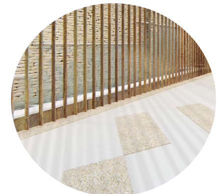
Edge Detail of Concrete and Granite Floors
