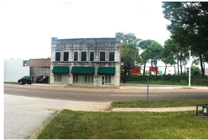
1. Masonry Building on Union Avenue
