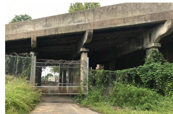
6. Bridge at Monroe Avenue
