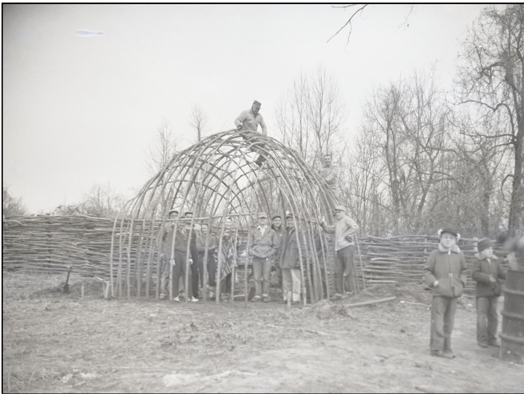
Figure 27b. Completed construction (pre-thatching) of the same open corner, bent pole structure at Chucalissa in 1955. Courtesy of the C. H. Nash Museum at Chucalissa.
