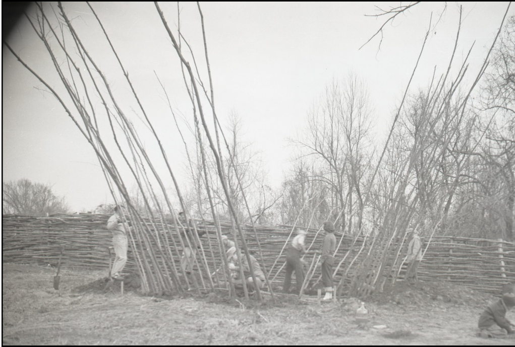
Figure 27a. Beginning of construction of an open corner, bent pole structure at Chucalissa in 1955. Courtesy of the C. H. Nash Museum at Chucalissa.
