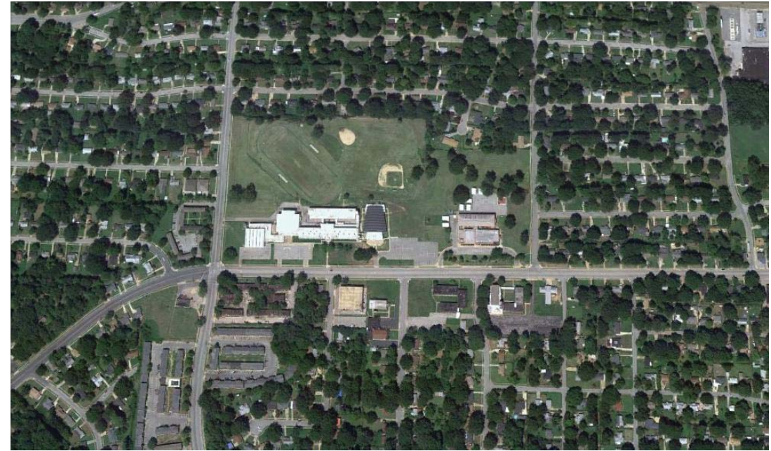
FIGURE 1. Frayser Aerial View, from Google Earth, 26 August 2011.
