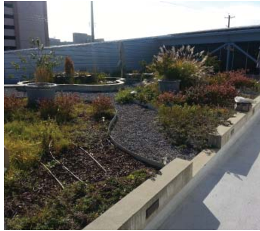
FIGURE 22. Roof Garden, by Victor Robinson, 2013.
