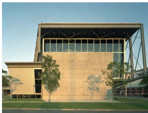
FIGURE 31. Western Gathering Space, photo from buildingstudio.net, accessed 2013.
