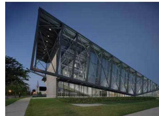
FIGURE 24. BRIDGES Southern Facade, photo from buildingstudio.net, accessed 2013.
