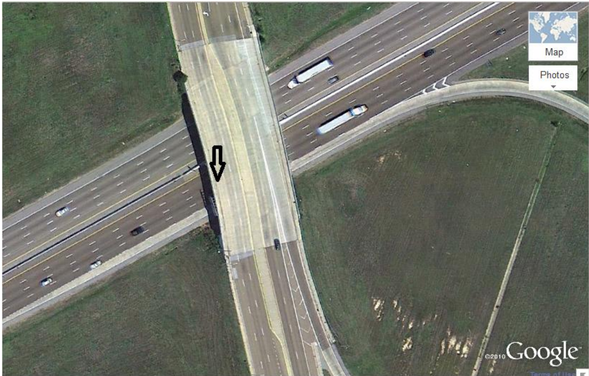
Figure 3. Location of the Appling Road Exit overpass bridge
