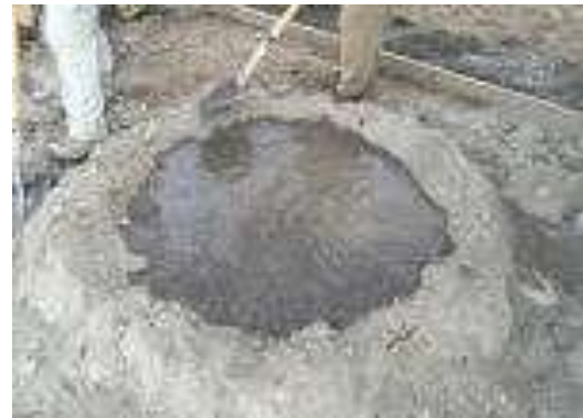
Fig. 2. Mixing of concrete
