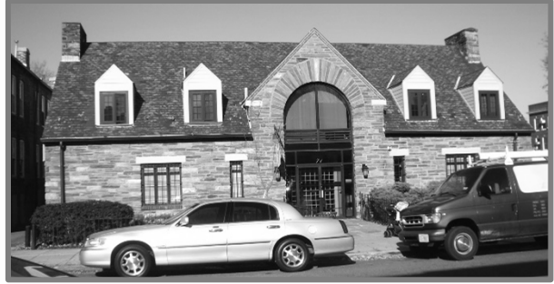
Former WARL shelter on O Street Photo by author
