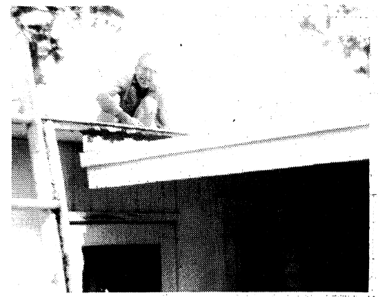
Poor old Doc! Emily puts him to work repairing a shed roof.
