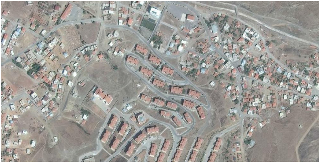
Figure B.48 Aerial view showing the relationship between the project and surrounding urban fabric
