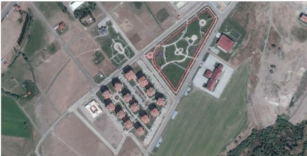
Figure B.18 Aerial view showing the relationship between the project and surrounding urban fabric
