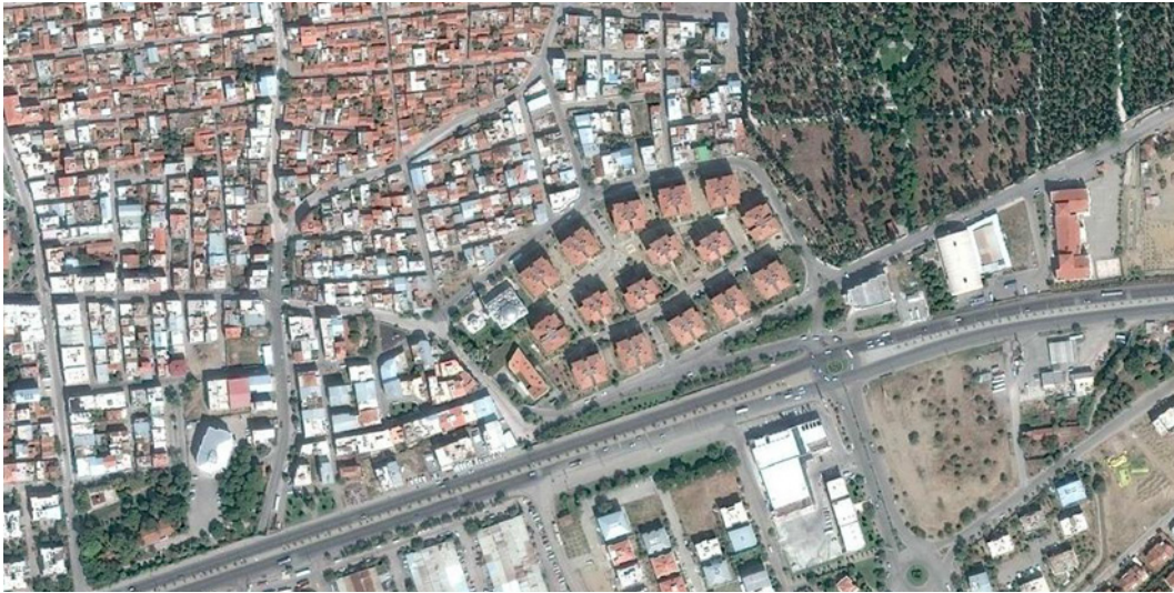
Figure B.58 Aerial view showing the relationship between the project and surrounding urban fabric
