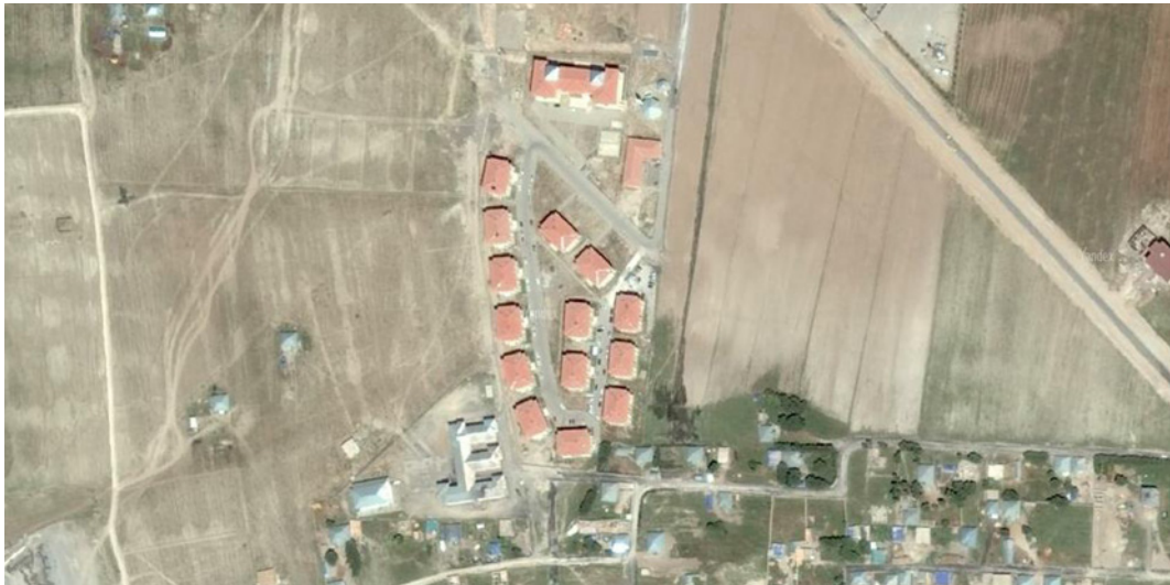
Figure B.12 Aerial view showing the relationship between the project and surrounding urban fabric
