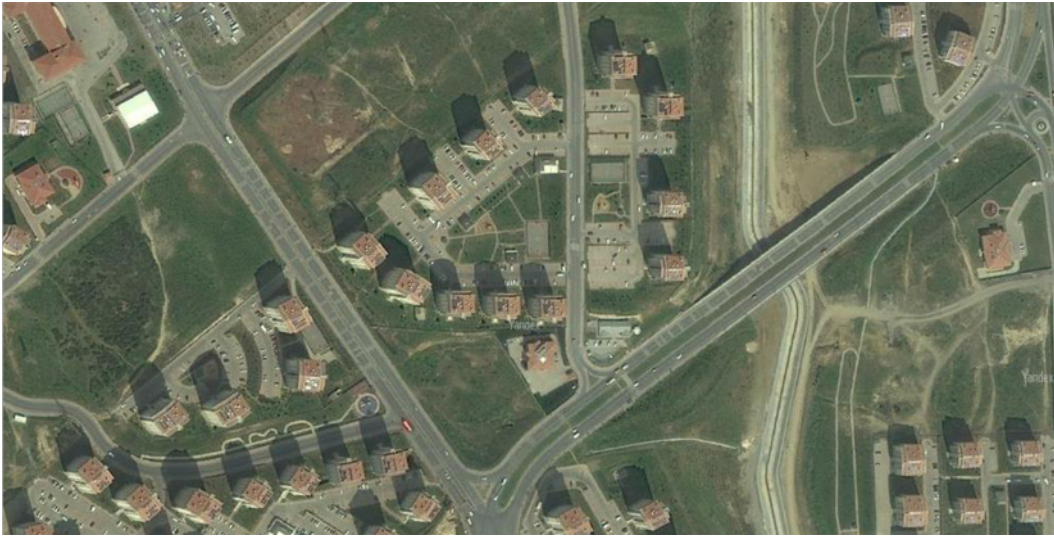
Figure B.46 Aerial view showing the relationship between the project and surrounding urban fabric
