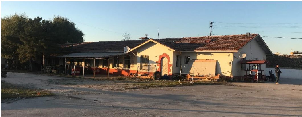
Figure 3.127. Meydan building (author, 2018)
