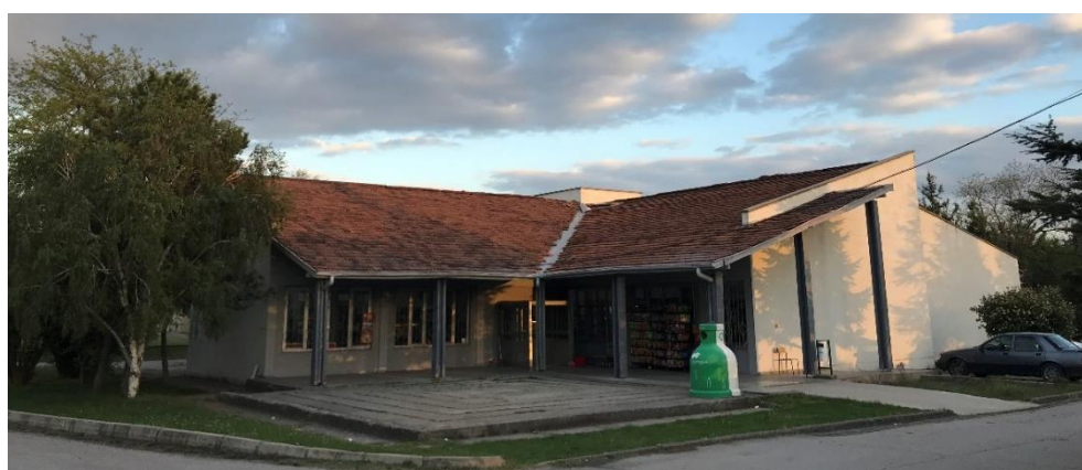
Figure 3.157. Canteen building (Author, 2018)
