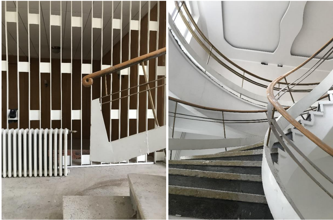
Figure 3.28. Guest-house, details from the original stairsteps (Author, 2017)
