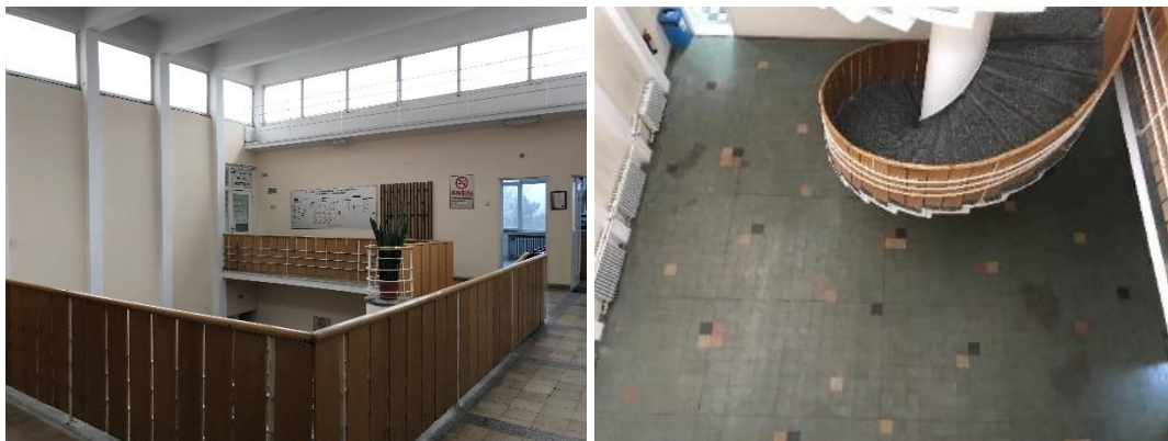
Figure 3.123. ceiling windows, Original floor tile (author, 2017)
