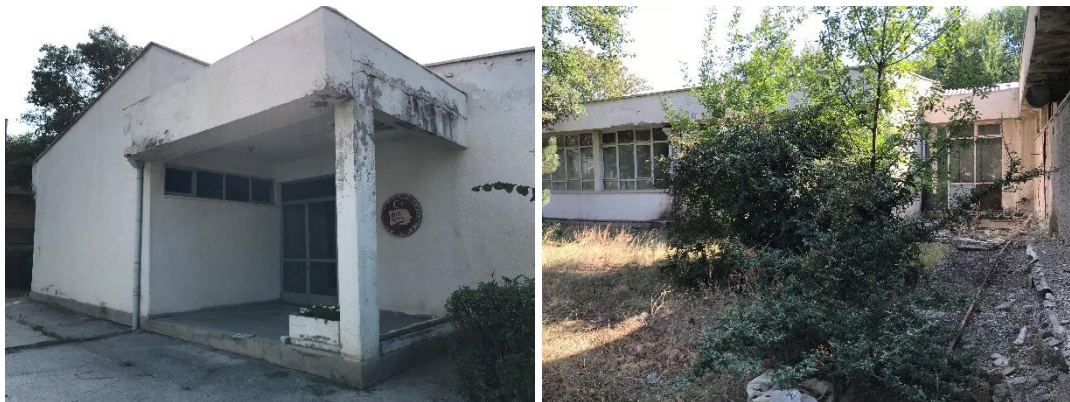
Figure 4.5. left: Confectionery Plant entrance, right: courtyard of the Plant (author,2018).
