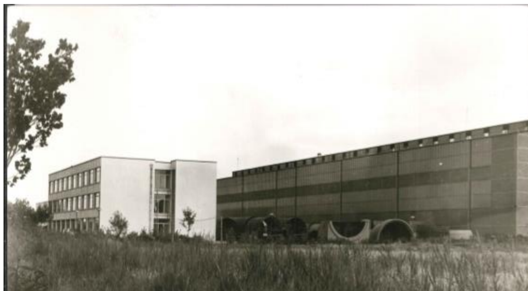
Figure 3.48. Ankara Machinery Factory Administrative Building and 1st Hall (archive of TSFAS)
