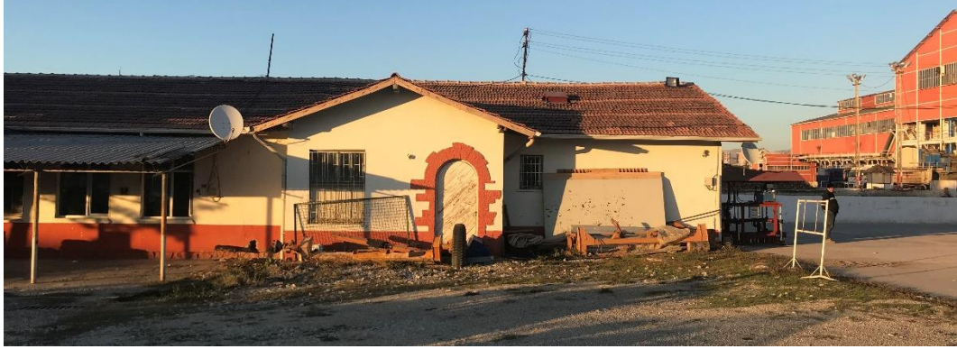
Figure 1.2. The archive and agricultural workshop share the same building in half. (author, 2018)
