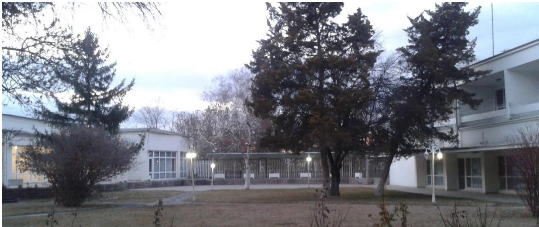
Figure 3.29. Pergola between the cinema-restaurant building (Author, 2017)
