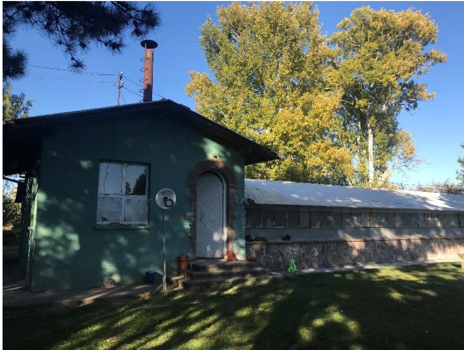
Figure 3.154. Workers' rest room and greenhouse (Author, 2018)
