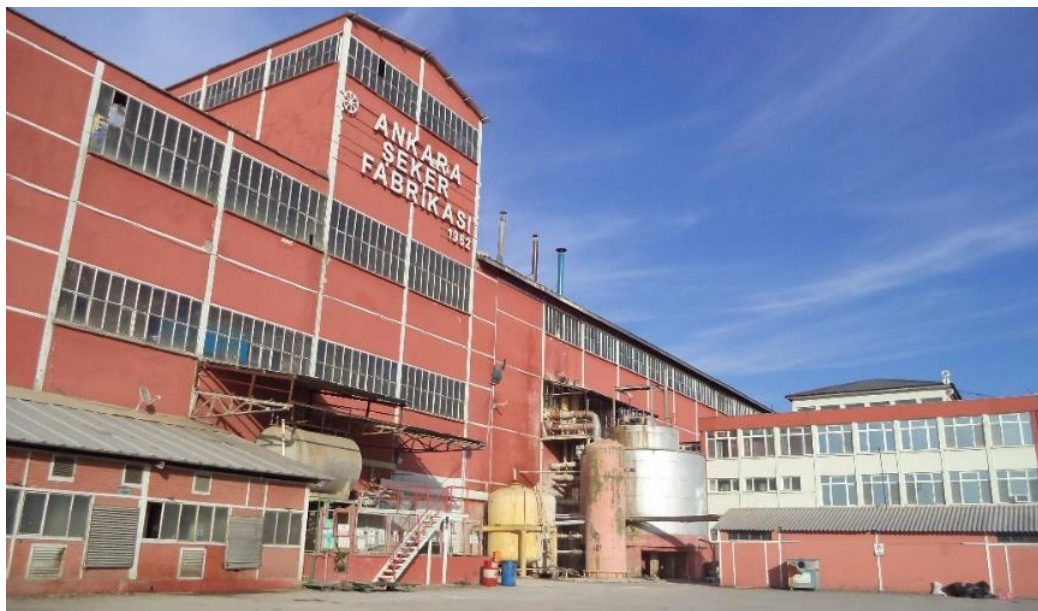
Figure 3.119. Sugar Factory Main Building and Office building (Author, 2017)
