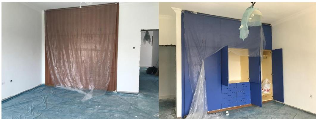
Figure 4.13. Renovation of stabile furnitures of the lodging
