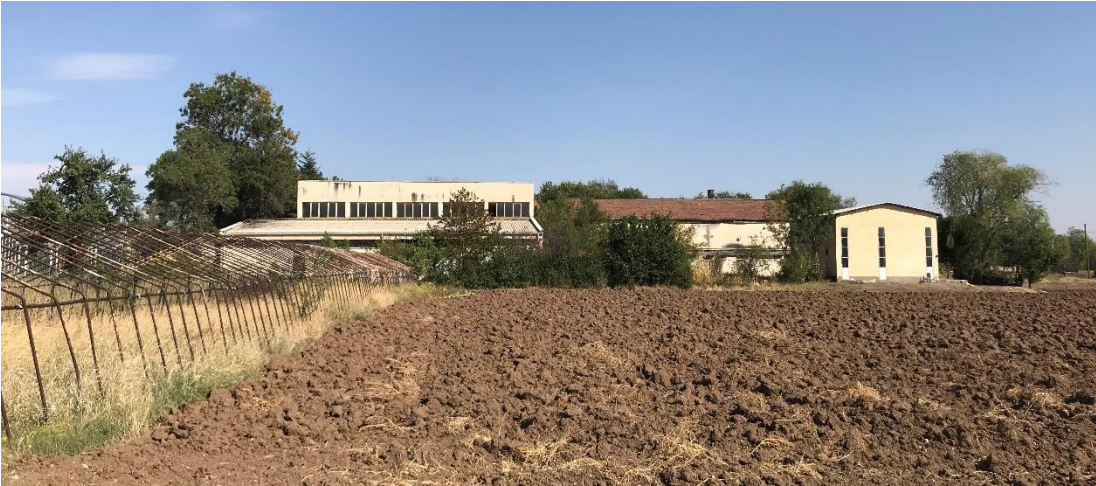
Figure 3.165. East facade of the Confectionary Production Facility (Author,2018)
