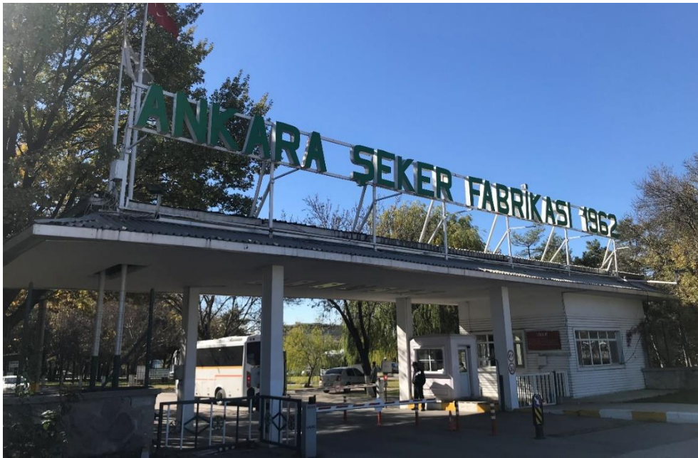
Figure 3.112. Benzinlik Gate, main entrance (author, 2018)
