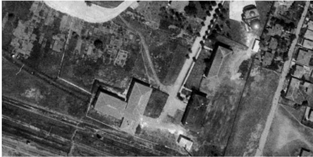
Figure 3.81. New workers pavillion (1988 aerial photo, general Command of Map)
