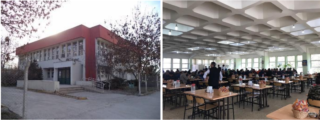
Figure 3.129. Left: dining hall; right: the hall in upperstairs (author, 2018)
