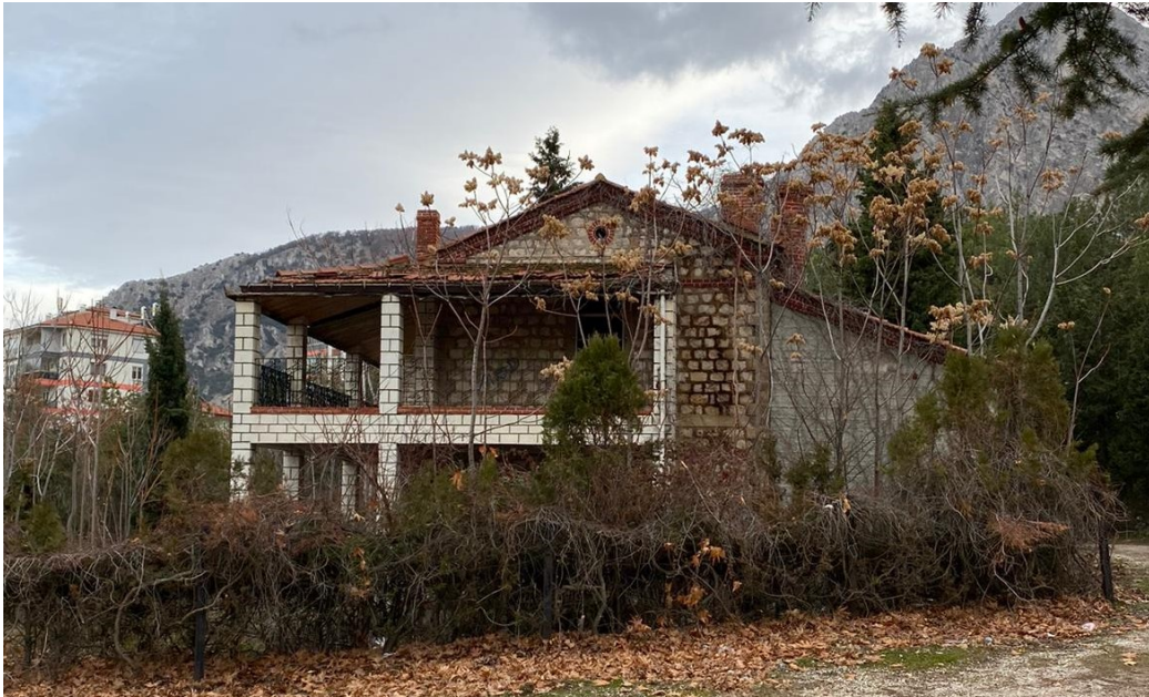
Figure 4.53: Photo of Guest House (Sinan, 2019)
