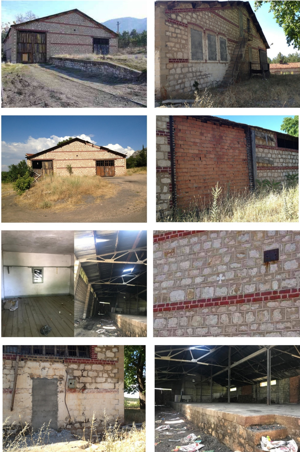
Figure 4.66: Photos of Warehouse Building (Sinan, 2019)
