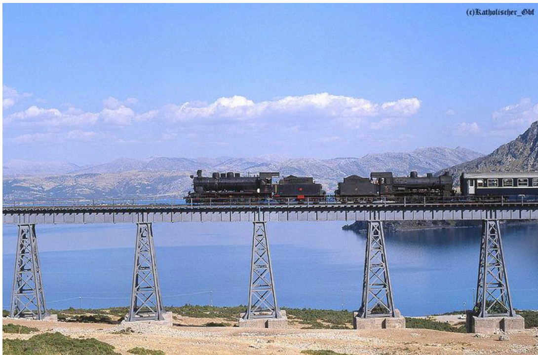
Figure 4.88: A Historical Photo of Bridge (Eğirdir Akin Newspaper Archive)
