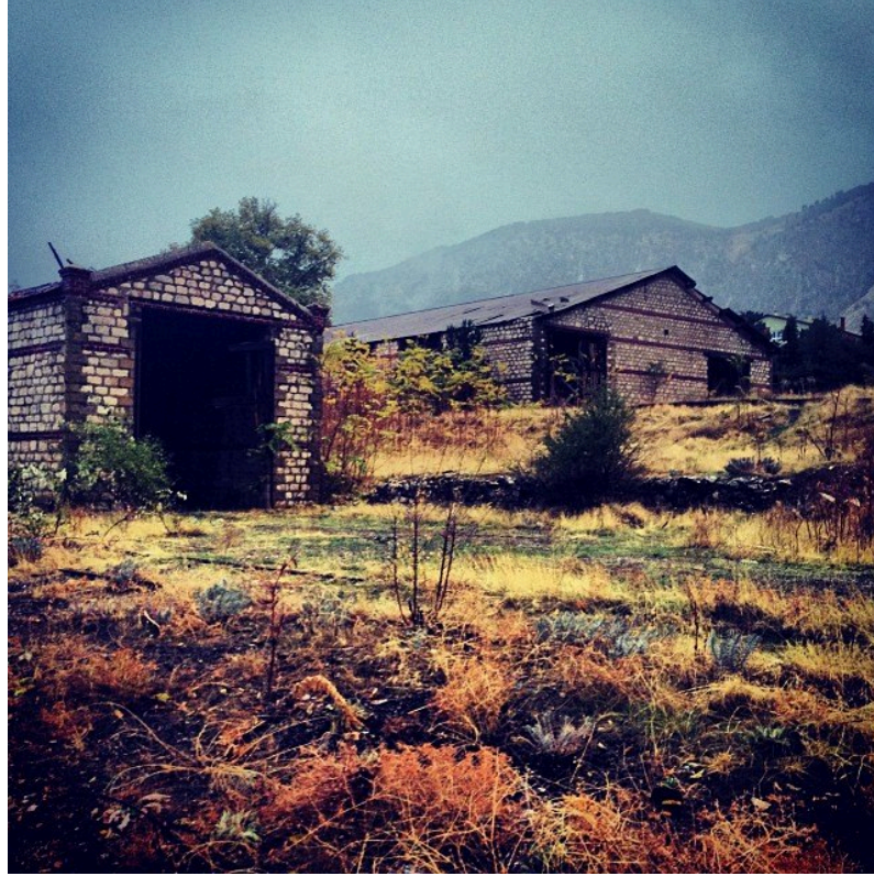
Figure 4.70: Photo of Cer Building (Sinan, 2019)
