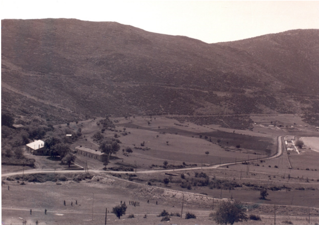
Figure 4.15: Station Area in 1970s. (Eğirdir Akin Newspaper Archive)
