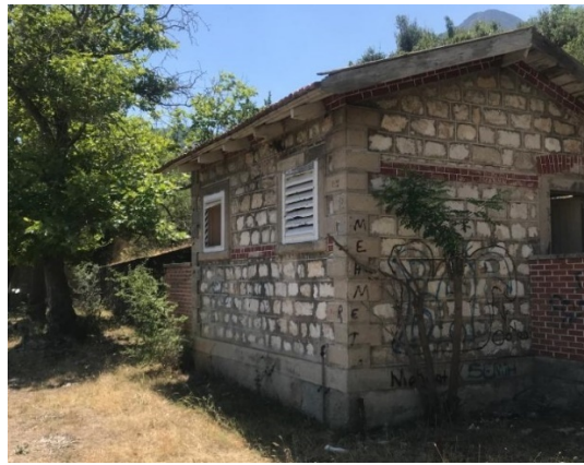
Figure 4.83: Photo of Toilet (Sinan, 2019)
