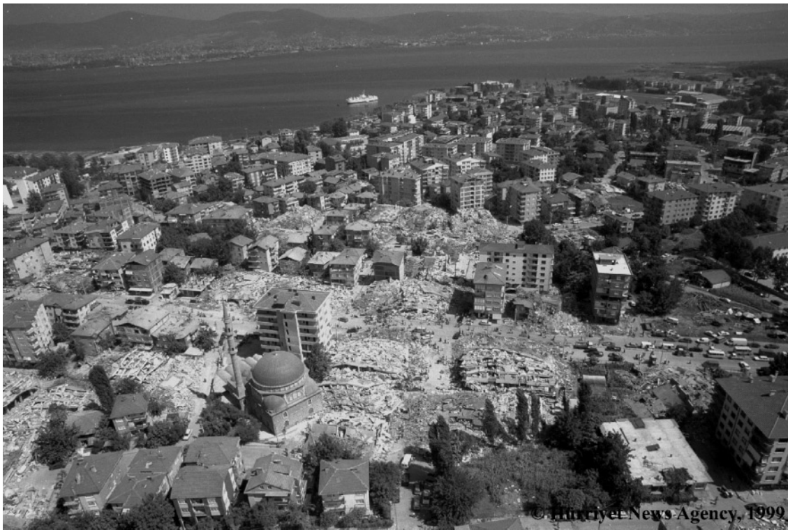
Figure 2. Aerial view of central area of Gölcük. Construction practices limit the drift capacity of typical framed buildings that are usually weaker in the ground story. The result can be structural instability and excessive damage, including collapse.
