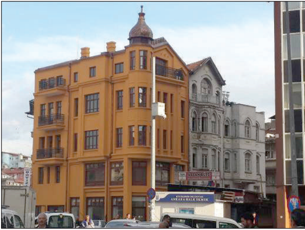
Figure 2A. Erzurum Hotel (Alsancak Street, No: 15), Avrupa Hotel (Susam Street, No: 8) and its addition (Susam and Tahtakale Streets). View from Hal Square. Date: 1916/1917-1920s.
