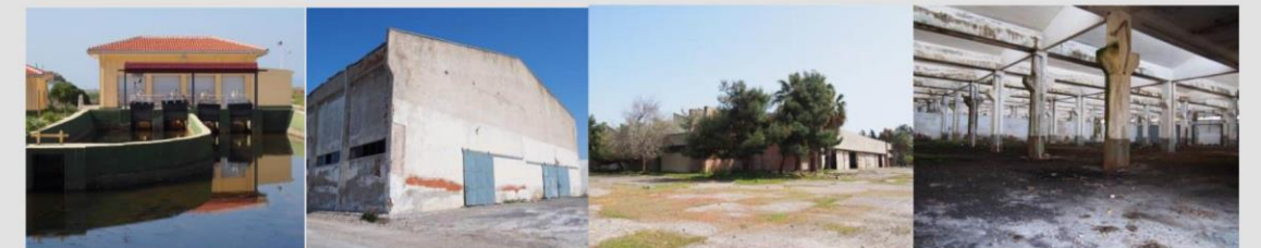
New Pump Station (3), Machine Hangar (15), Ateliers Building exterior and Interior (119)
