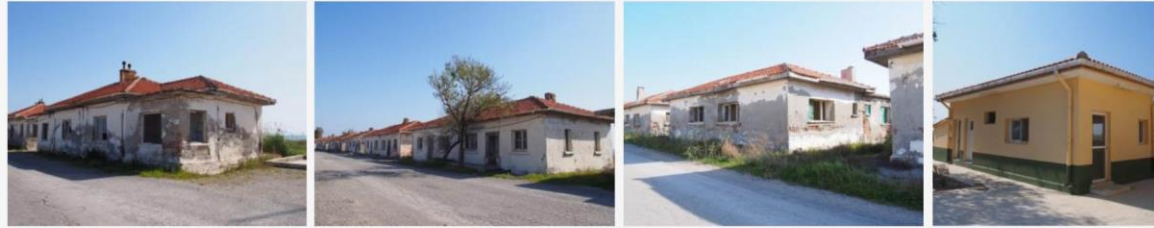
Lodging Type 4(38, 39, 40, 41), Lodging Type 5(42, 43, 44, 45,46,47), Lodging Type 6(49, 54, 55,56,57,58,59,60,61), Locker Rooms and Watchbox(4)
