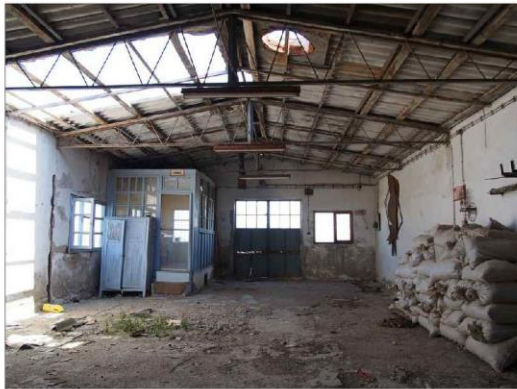
Manager's office (1) and rail atelier (2)
