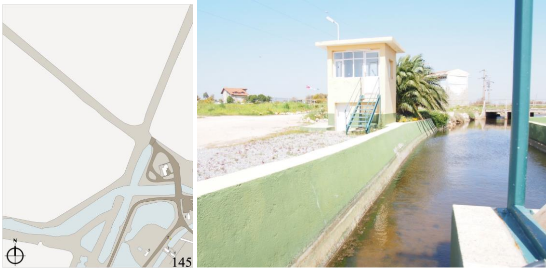
Figure 99 Site plan and southwestern facade of the watchbox (Author, April 2016)
