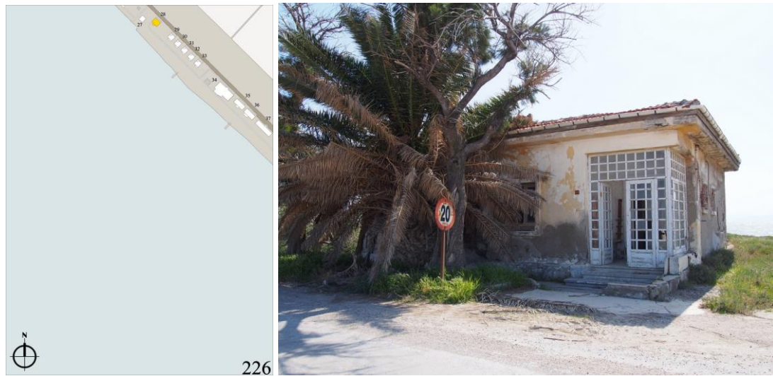
Figure 112 Site plan and northeastern facade of the lodging type 1 (Author, April 2016)
