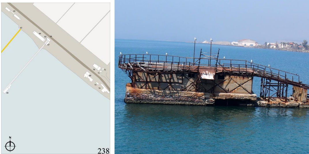
Figure 123 Site plan and the northwestern facade of the port 1 (Author, April 2016)
