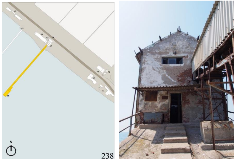
Figure 125 Site plan and the northeastern facade of the port building 2 (Author, April 2016)
