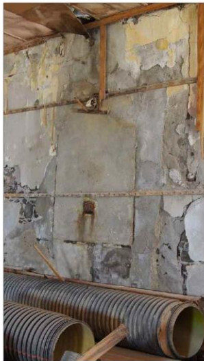
Closed window opening
