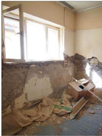
Room wall construction (6)
