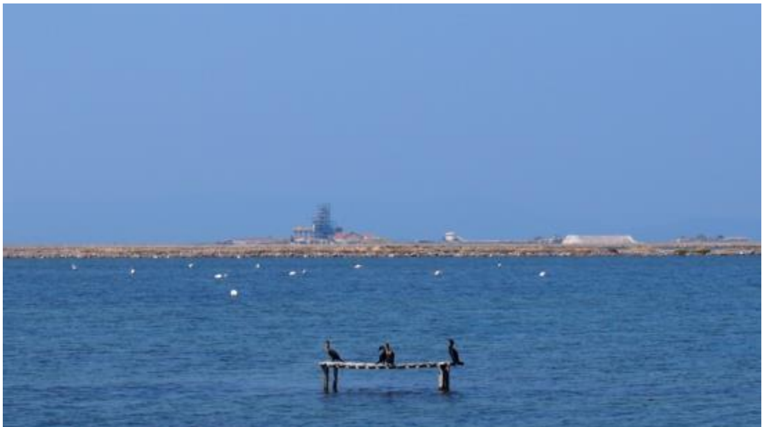
Figure 87 Bird nest in one of the salt pans, salt washing plant and the technical building on the background (Author, April 2016)
