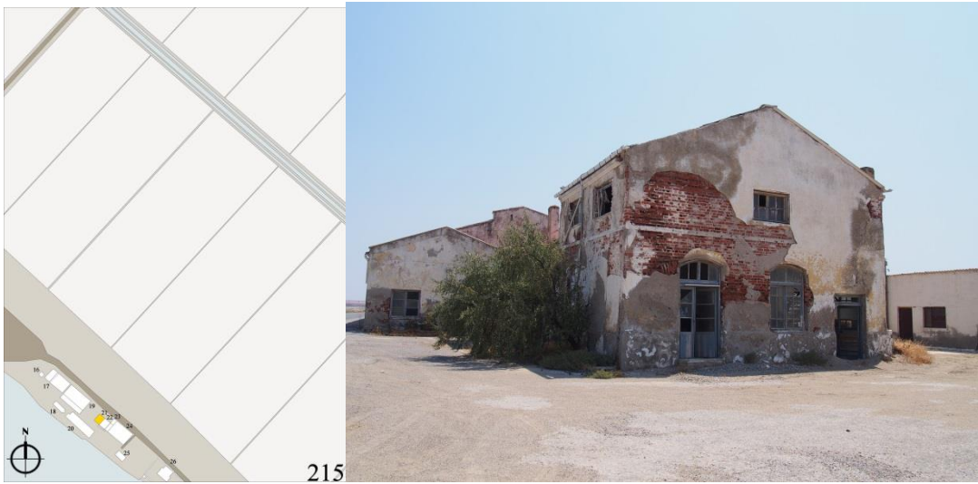
Figure 107 Site plan and view from the northern corner of the house? 1 (Author, April 2016)
