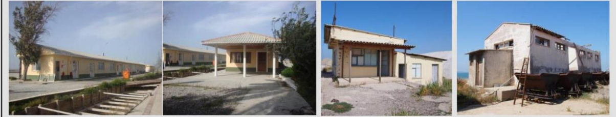
Ateliers (9, 10, 85,87), Administration (11), Old scale (13), Toilets (18)
