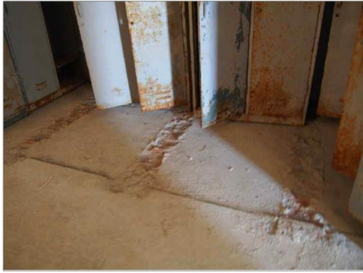
Demolished basin platforms (2)
