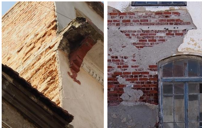
Figure 95 A house in Kemeraltı, bricks with cavities having solid brick dimensions and similar brick in Çamaltı (Author, April 2016)
