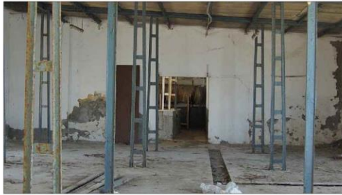
Refectory (3) to Kitchen (4)
