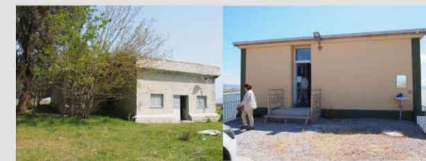
Water Tanks(78,125) , Second Pump Station(7)
