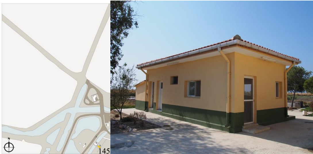
Figure 100 Site plan and view from the northern corner of the locker rooms and watchbox (Author, April 2016)
