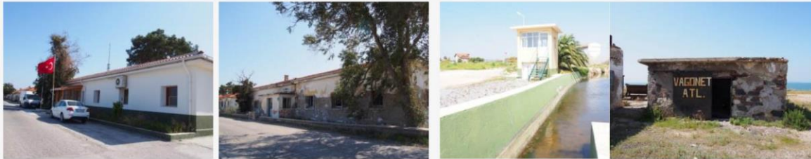
Infirmary(37), School(34), Watchbox(2), Small Storage (16)
