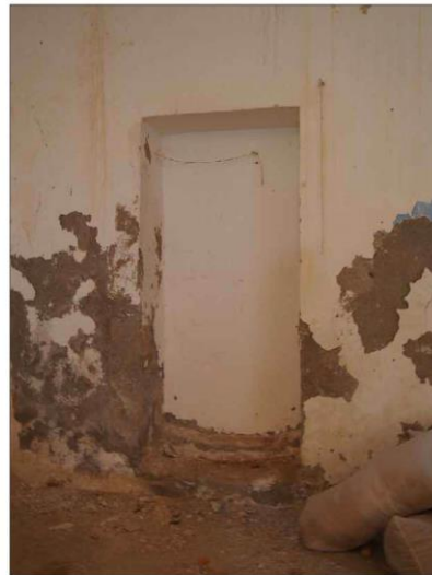
One of the closed door openings on screen wall
