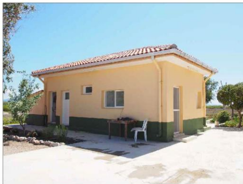
Entrance to Wc (4-5)
