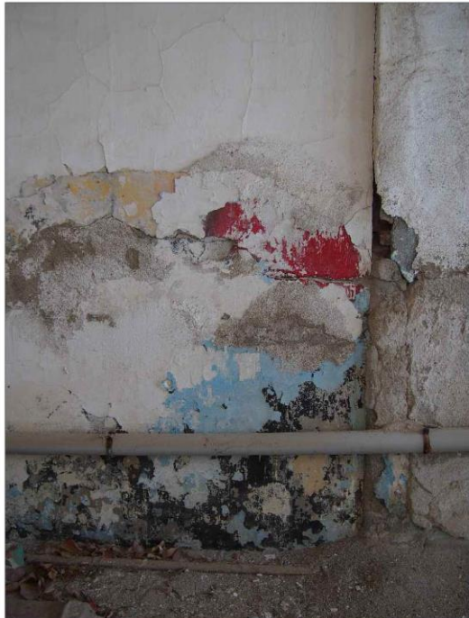
Connection between two walls
