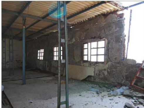
Refectory and demolished wall (2)
