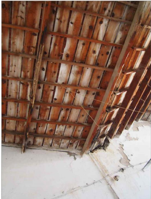
Connection between two roofs
