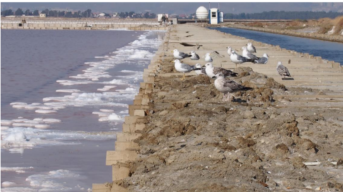
Figure 93 Wooden border filled with clay (Author, August 2016)
