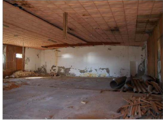
Cinema hall and screen wall (1)
