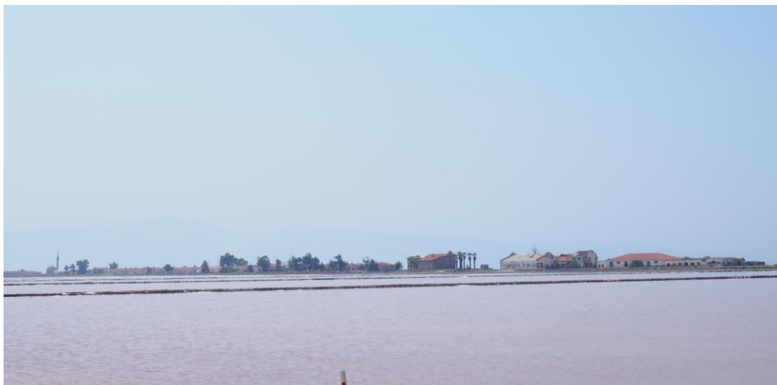
Figure 136 Abandoned buildings and the crystallisation pools (Author, August 2016)
