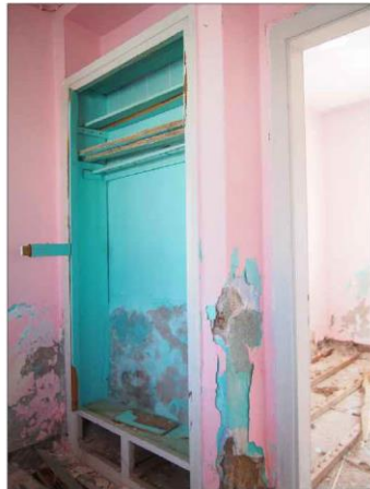
Room closet and 6.room (7)
