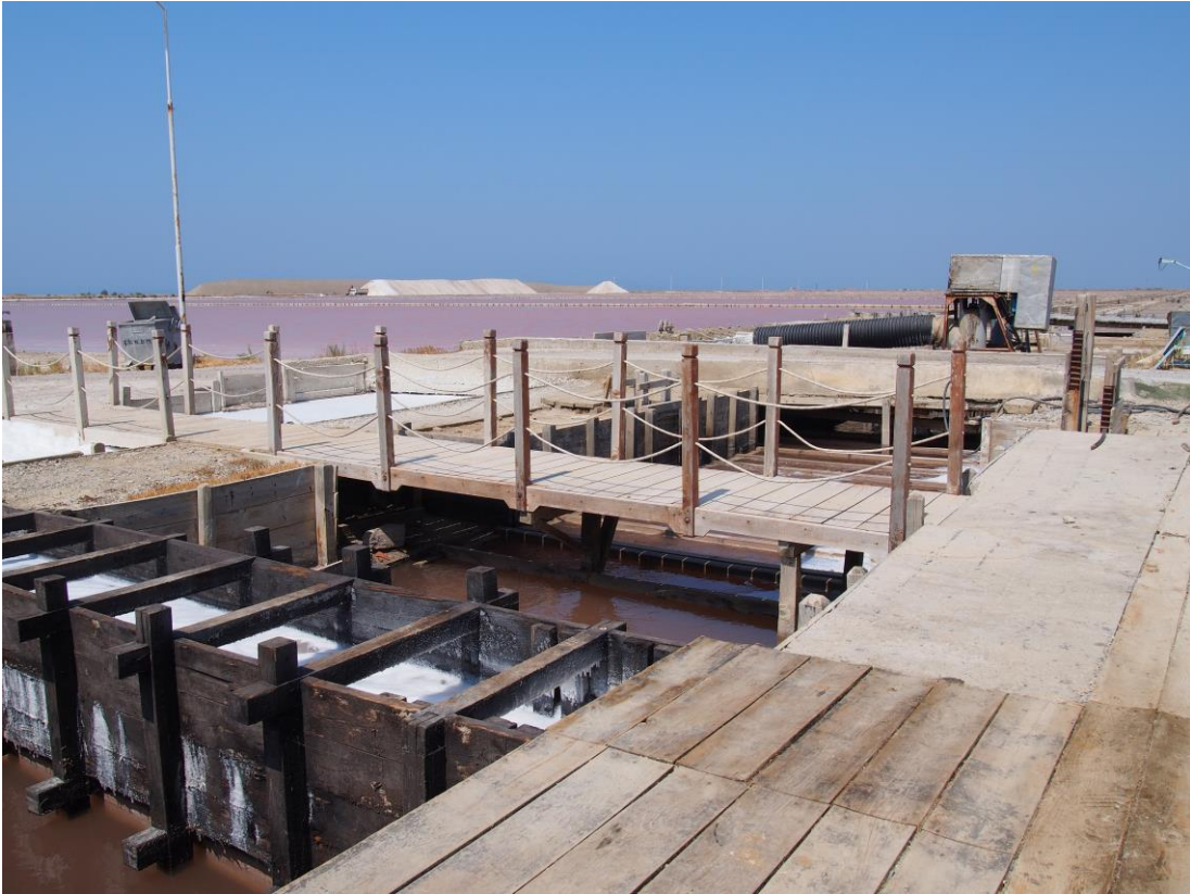
Figure 92 Water channels built with wood (Author, August 2016)
