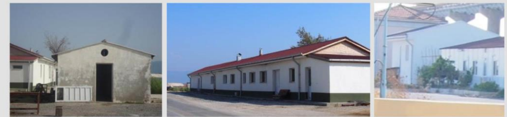
Toilets (73, 100), Refectory (74), Laboratory Storage (82)
