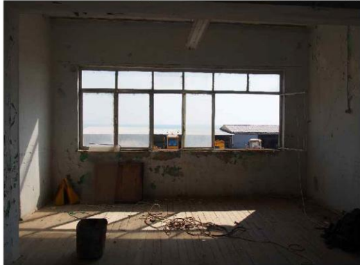
Room and closed balcony (17)
