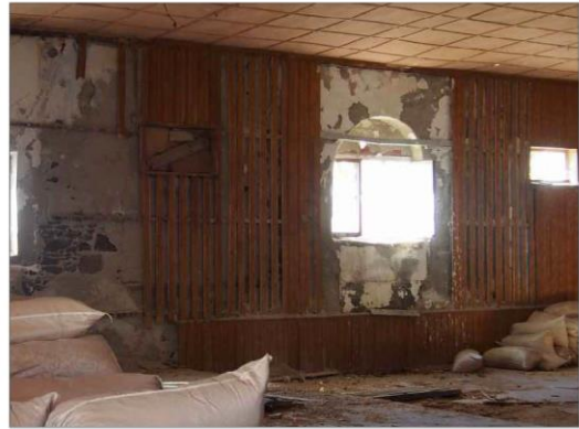
Cinema hall walls and windows
