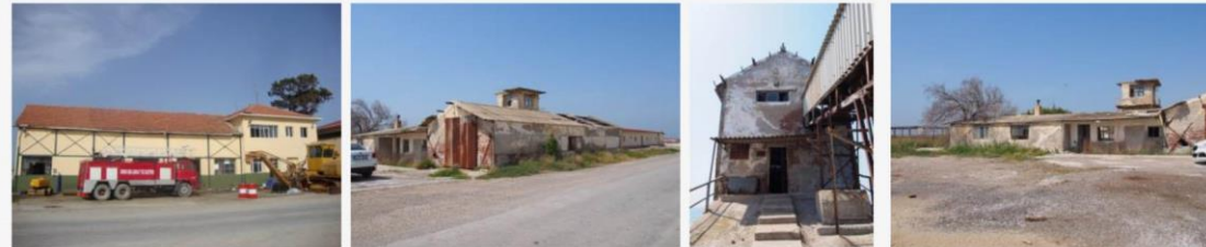
Old Power Plant(70), Port 2 building 1(66), Port 2 Building 2(68), Office(67)
