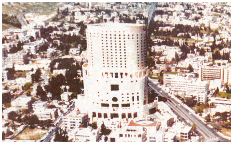
Figure 11. Le Royal building. (Greater Amman Municipality, 2007).
