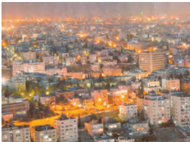
Figure 12. Examples of high rise building during 1970s at Amman. (Greater Amman Municipality, 2007).
