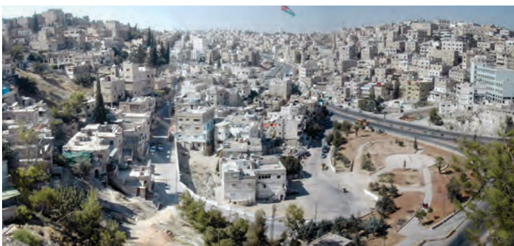
Figure 22. Northern section of Amman skyline. (Al-Ghazalah, 2007).
